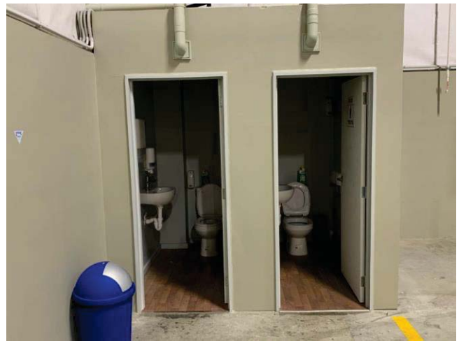
Toilets within Warehouse
