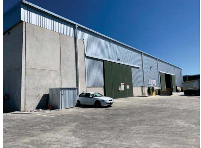
Coolpak Coolstores (Building 2)
