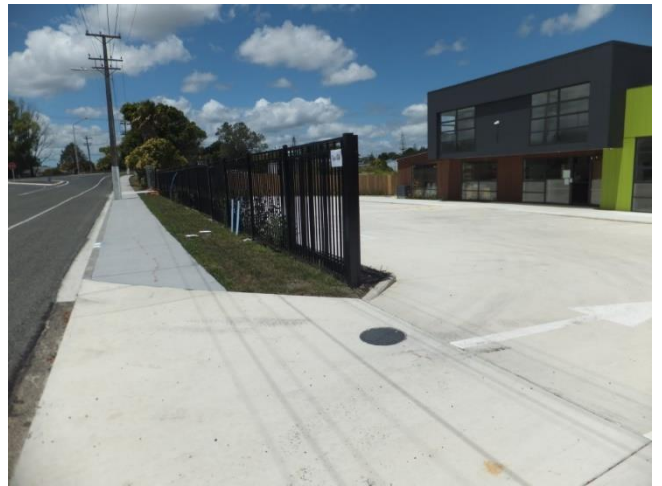
Car park and front boundary
