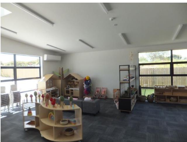
LED strip lighting
