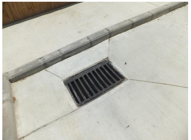
Stormwater drainage gully
