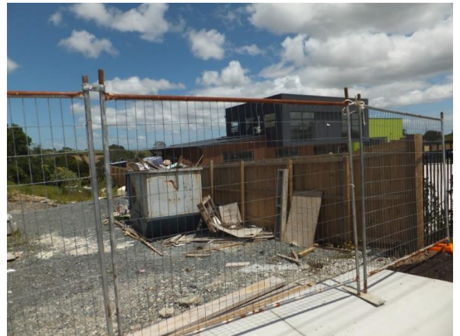
4. Air con unit visible above ground floor roof
