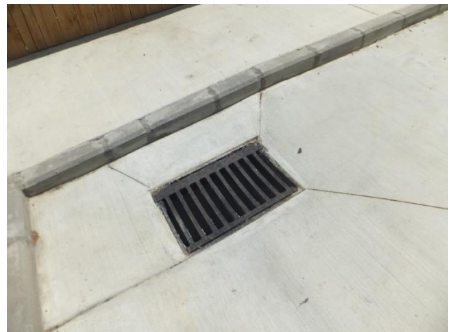
Stormwater drainage gully
