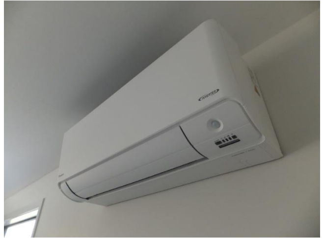
Indoor split system Air-Conditioning unit
