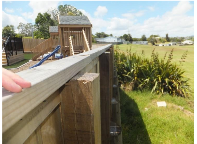
Retaining wall to rear boundary
