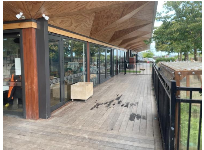
Covered timber deck and adjoining playground development
