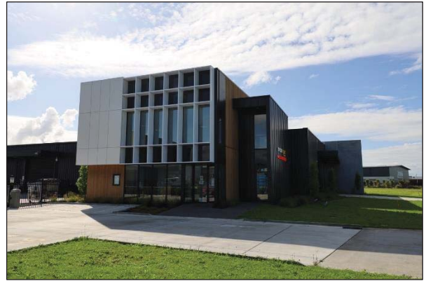
Ground and first floor office
