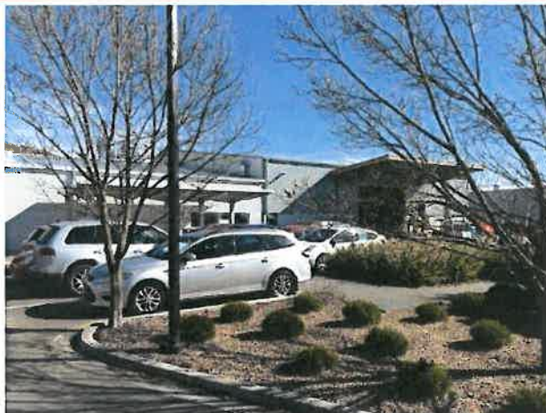
Warehouse and Canopy
