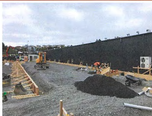
Existing warehouse and new office slab under construction adjacent
