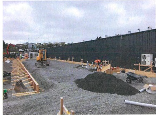
Existing warehouse and new office slab under construction adjacent
