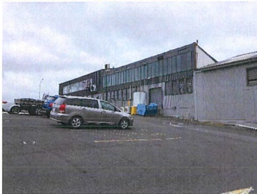
Existing Office- to be demolished
