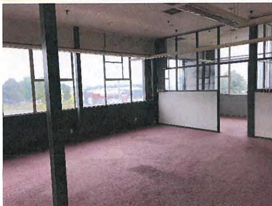
First Floor Office - Vacant
