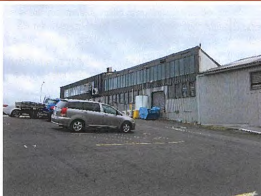
Existing Office- to be demolished
