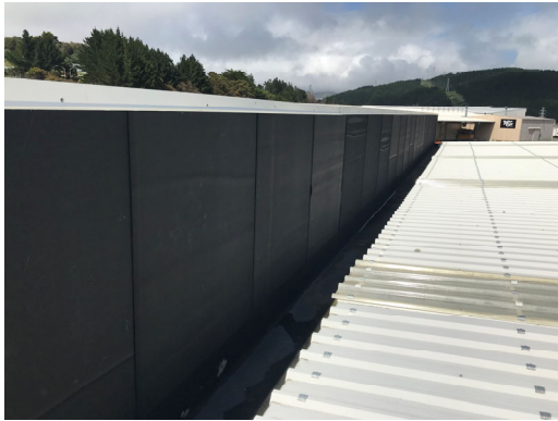
1.7. Building 2 – Membrane Flashings
