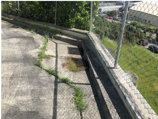
1.55. Evidence of subsidence to north east corner of site
