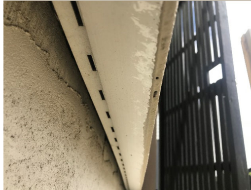
1.7. Weep holes visible to underside of panel
