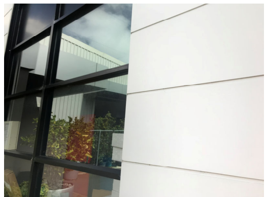
1.36. Building 2 – Fibre cement sheets/aluminium windows
