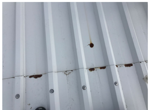
1.18. Building 1 – Poor Overlap Detail
