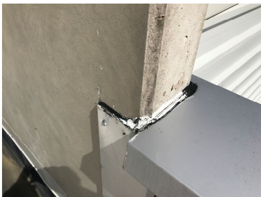
1.11. Building 2 – Poor Detailing
