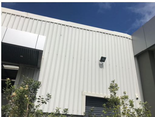
1.35. Building 2 – External Cladding
