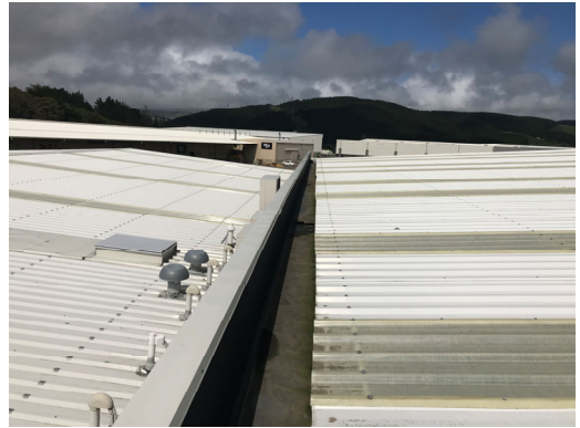
1.14. Building 1 – Membrane Gutters
