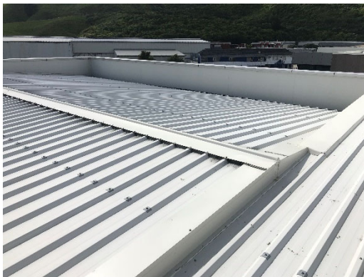
1.5. Poor detailing to office/warehouse junction
