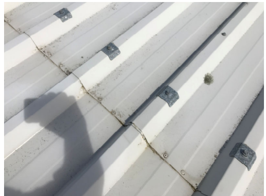
1.10. Building 2 – Poor Overlap Detail
