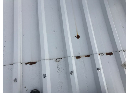
1.4. Corrosion along length of overlap joint
