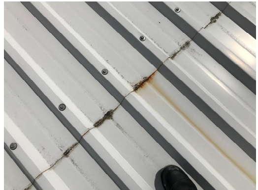
1.16. Building 1 – Poor Overlap Detail
