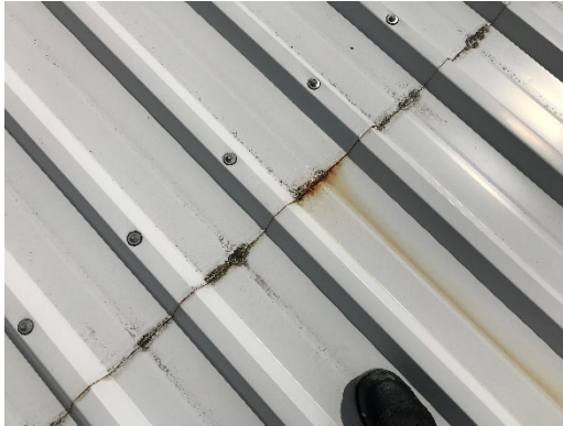
1.3. Corrosion along length of overlap joint
