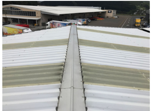
1.4. Building 3 – Ridge Flashings
