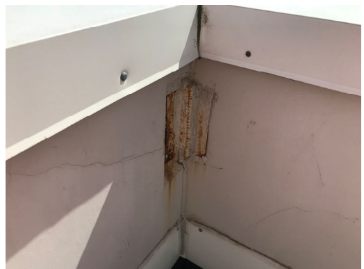
1.6. Building 3 – Corroding Plate
