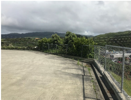
1.8. Railings above retaining wall noted to be falling outwards
