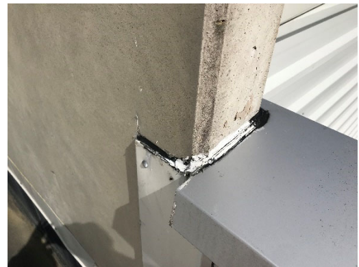
1.6. Poor detailing to parapet/tilt slab junction
