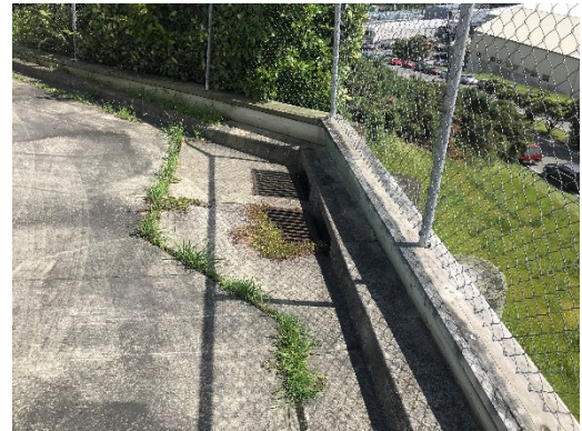
1.9. Grass growth occurring where joints are opening up
