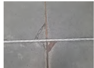
46. Cracking observed to the concrete slab flooring of the warehouse, adjacent to movement joints within extended section of warehouse.
