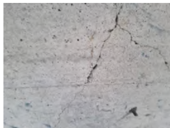
18. Cracking to the northeast panels (beneath the canopy) is wider to some areas.
