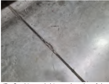
47. Cracking and chips to the edge of the concrete floor adjacent to the control joint.
