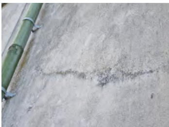
17. Localised spalling of panels adjacent to cracking and concrete infills around anchors in the panels to the southwest.
