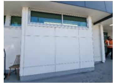
28. Example of single glazed window joinery.
