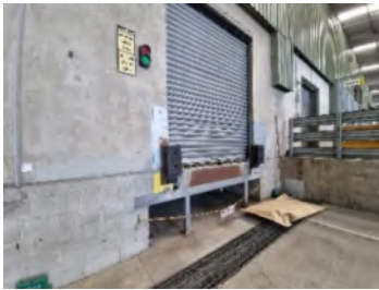
26. Example of dock roller shutter door and barriers.
