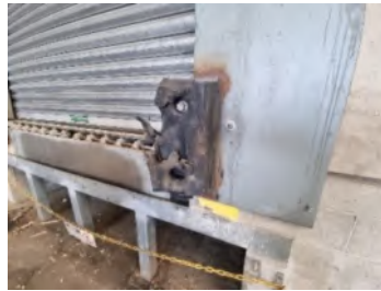
27. Deterioration of the rubber buffers.
