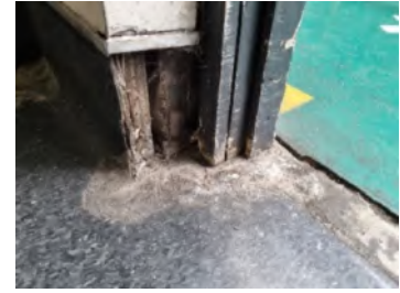
34. Isolated area of damage wall framing and lining adjacent to warehouse door between toilet corridor and warehouse.
