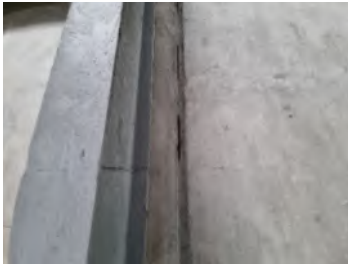
35. Openings within the flexible sealant between panels.
