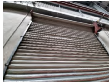
42. Typical view of roller shutter doors from interior. Doors are in a reasonable condition.
