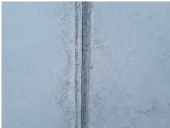
14. Seals to the panel junctions along the southeast wall have deteriorated and splitting was observed within the exterior flexible seal across the elevation.
