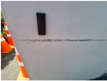
23. Deterioration of the cladding and painted finish at the horizontal expressed joint of the cladding.
