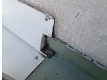
12. Flashings to the perimeter of the roof have not been chased into the adjoining concrete panels and rely on sealant for weathertightness. Flashings are of different style resulting in openings at flashing junctions.
