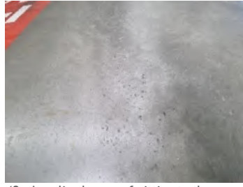
48. Localised areas of pitting to the surface of the concrete slabs within the warehouse (both the original and extended areas of the warehouse).
