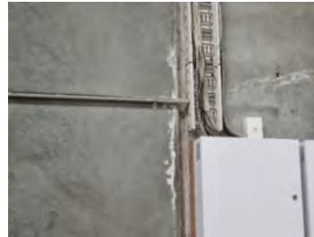
39. Hairline cracking and efflorescence surrounding cracks within pre-cast concrete panels.
