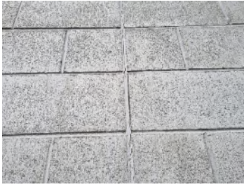
20. Splitting to the flexible seal along the control joint within the northwest fire wall (external view).
