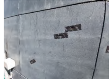
22. Impact damage to the fibre cement panels to the southeast elevation of office.
