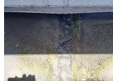
13. The butyl membrane to the internal gutter appears to have been patch repaired at laps. Staining indicates ponding may be occurring and that run off is not always directed towards outlets.
