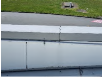
8. Chipping to the base of the fibre cement cladding to the parapet walls.
