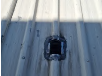
11. Boot flashings applied parallel to the sheet crests opposed to the preferred diagonal configuration. Sealant has been heavily applied around flashings and around service penetrations.
