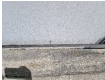
24. Cracking to the fibre cement panels of the security office, adjacent to fixings.
