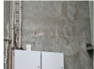
40. Hairline cracking and efflorescence surrounding cracks within pre-cast concrete panels.
