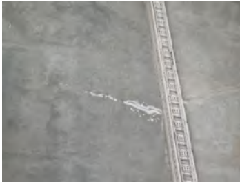
38. Hairline cracking and efflorescence surrounding cracks within pre-cast concrete panels.
