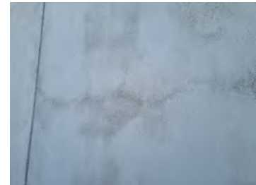
16. Hairline cracking to the exterior of panels observed to the southeast and southwest panels.
