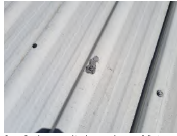
9. Sealant applied over the roof fixings.
