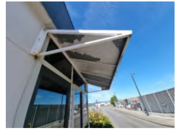
25. Corrosion of the metal framing and deterioration of the painted finish.
