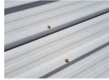
10. Corrosion of isolated fixings.
