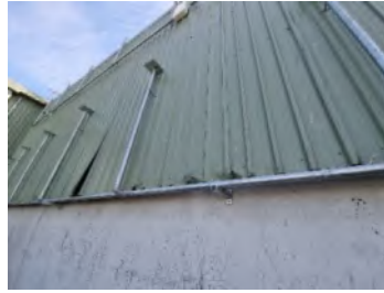
21. Detaching panel and impact damage to the base of panels to the partial southeast panels and length of the northeast panels.
