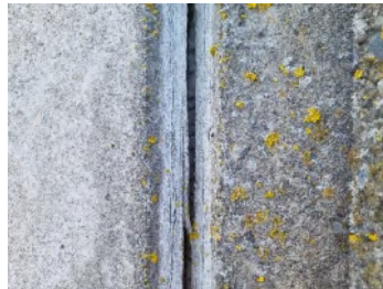
15. Seals to the panel junctions along the southwest wall have perished with splitting of the seals revealing the foam internal seal in numerous locations. Defect is evident across the elevation.
