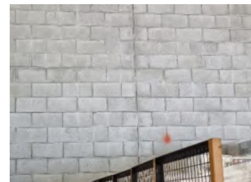
19. Splitting to the flexible seal along the control joint within the northwest fire wall (internal view).
