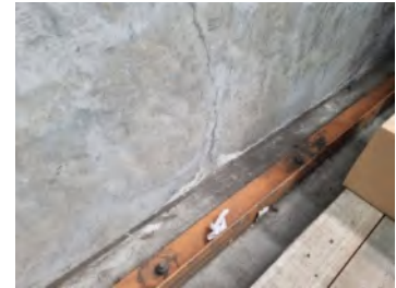
37. Hairline cracking and efflorescence surrounding cracks within pre-cast concrete panels.
