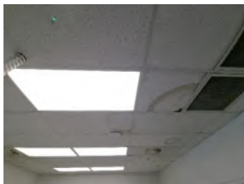
29. Moisture staining to the ceiling tiles of the ground floor office.
