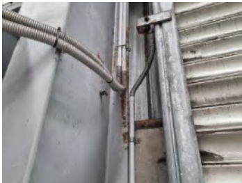
41. Isolated area of surface corrosion to the steel structure.
