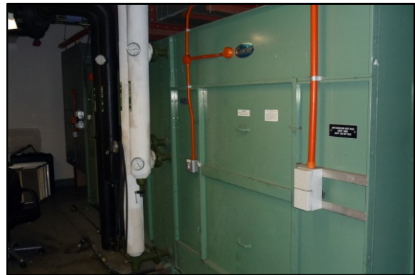
VAV Air Handling Unit
