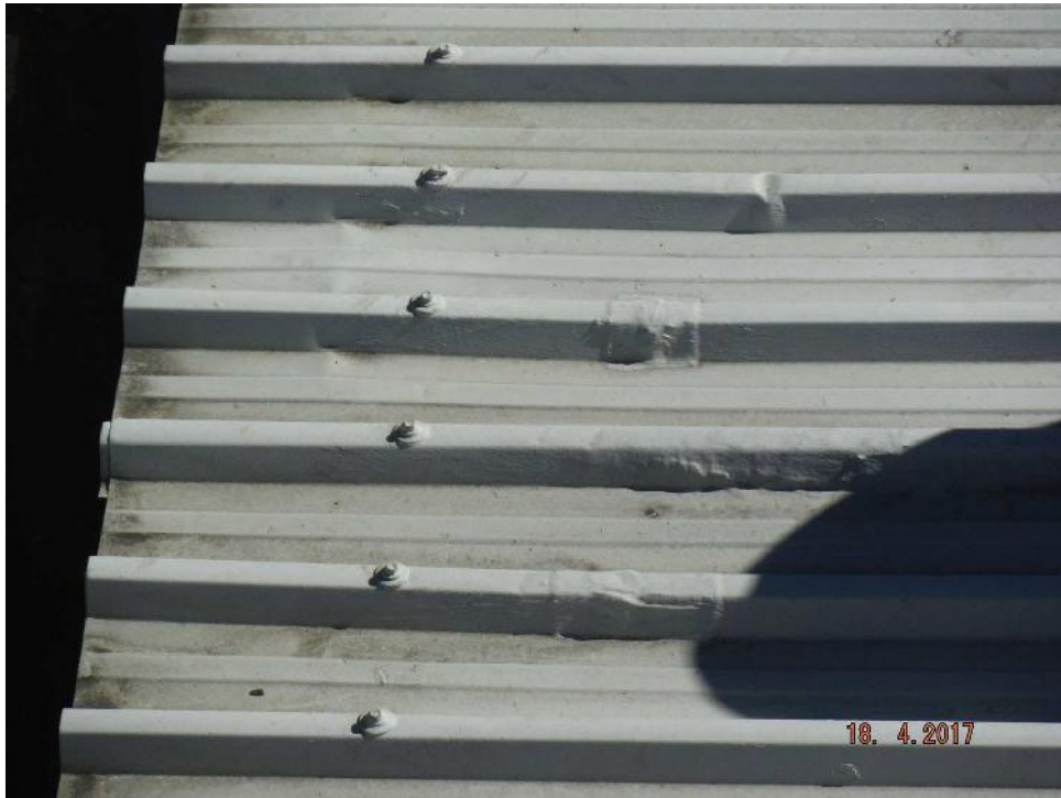
Photo 17: Patch repairs present to the lower roof.
