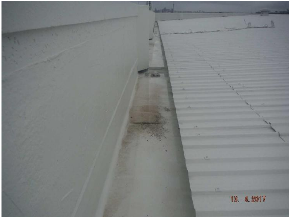
Photo 5: Gutters are formed from timber behind parapet walls and lined with butyl membrane.
