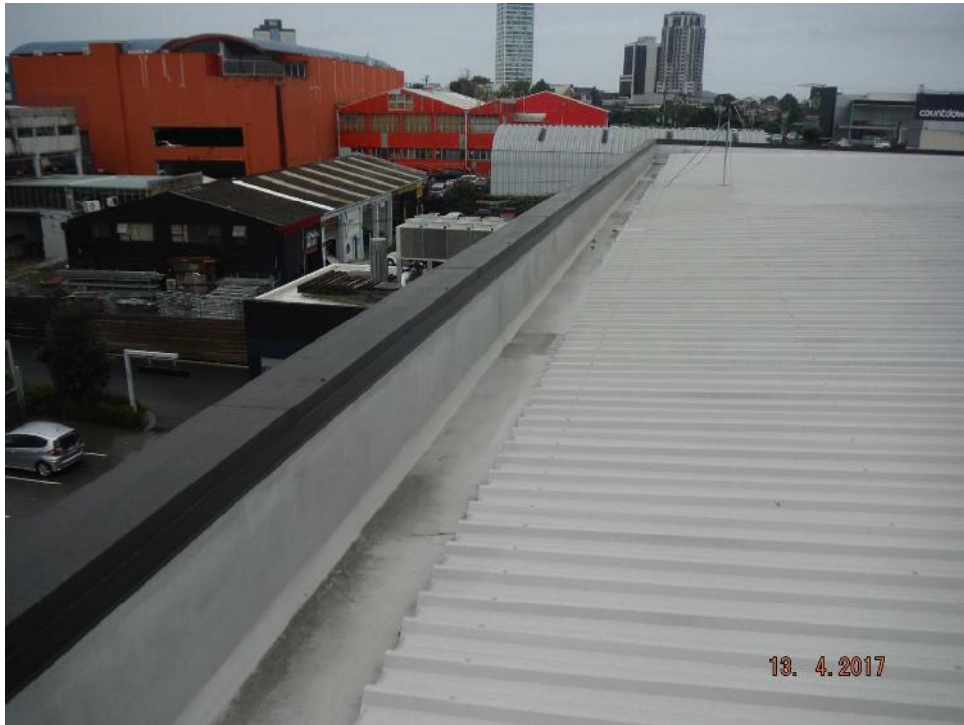
Photo 9: An elastomeric coating has been applied to membrane gutters.
