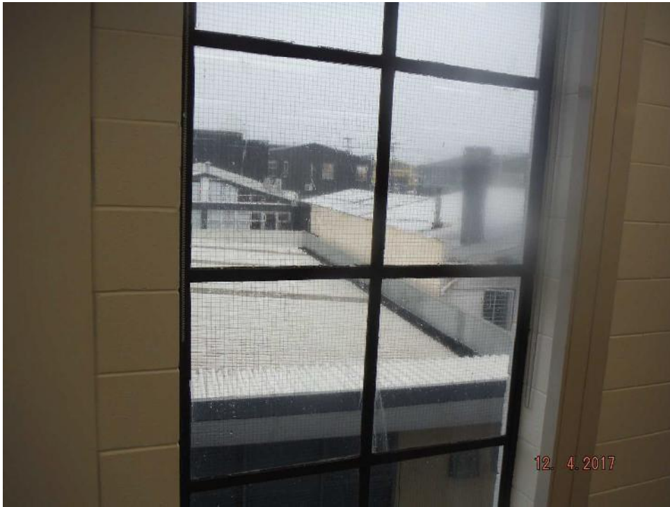
Photo 15: Steel framed windows to the rear elevation of level two are in a poor condition.
