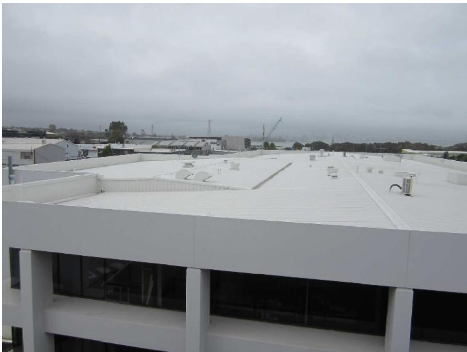
Photo 2: General view of the metal roof covering. The roof has been coated with a spray applied elastomeric coating.
