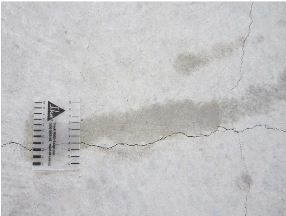
Photo 4: Numerous cracks are present to the concrete car park decks.
