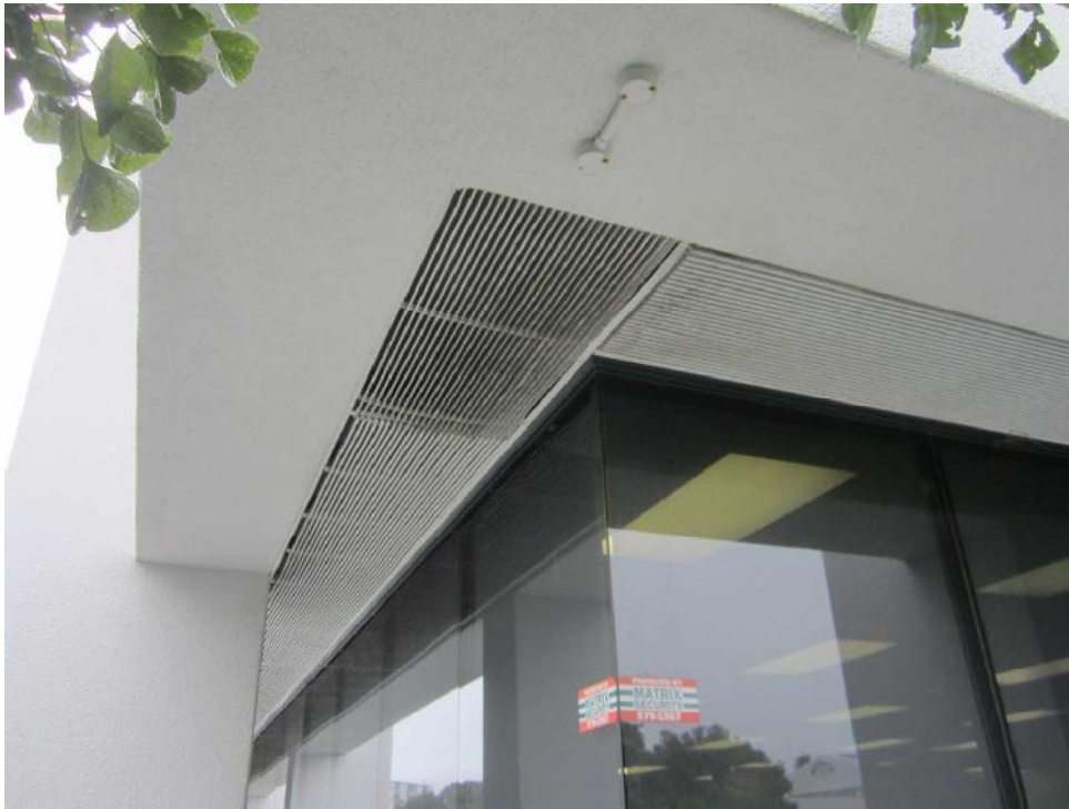
Photo 17: Soffit vents are installed to the perimeter of the building at each level. Grilles protecting the vents are missing in several locations.
