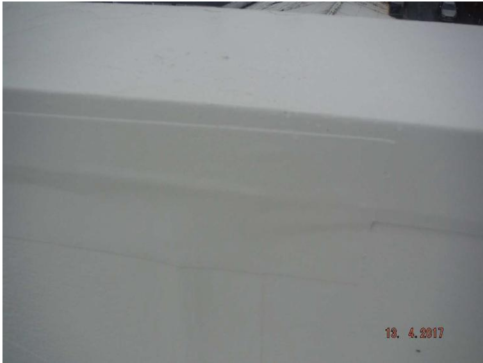
Photo 7: An elastomeric coating has been applied to parapet cappings. Evidence of previous patch repairs using flashing tape.
