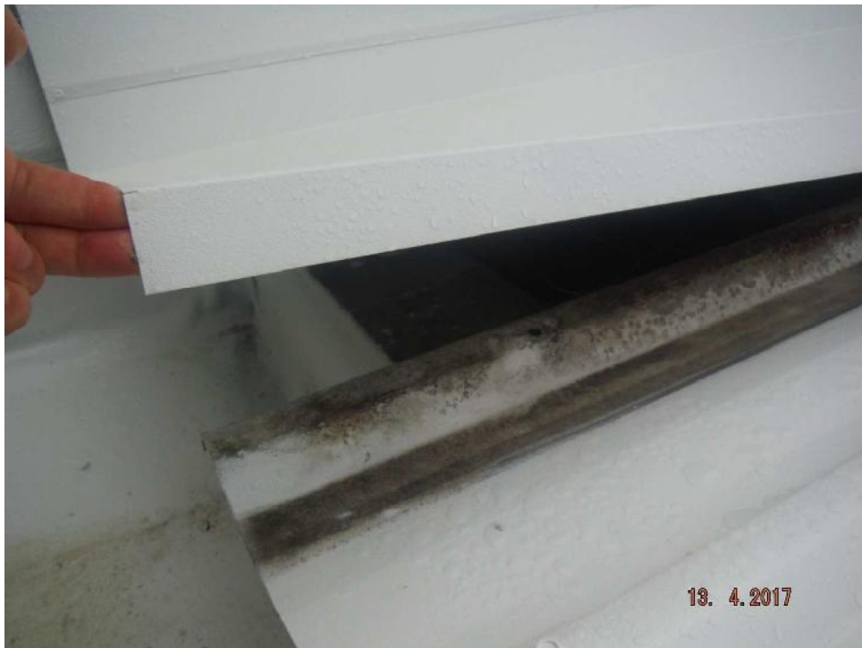
Photo 4: Several loose roof sheets and fixings were noted.
