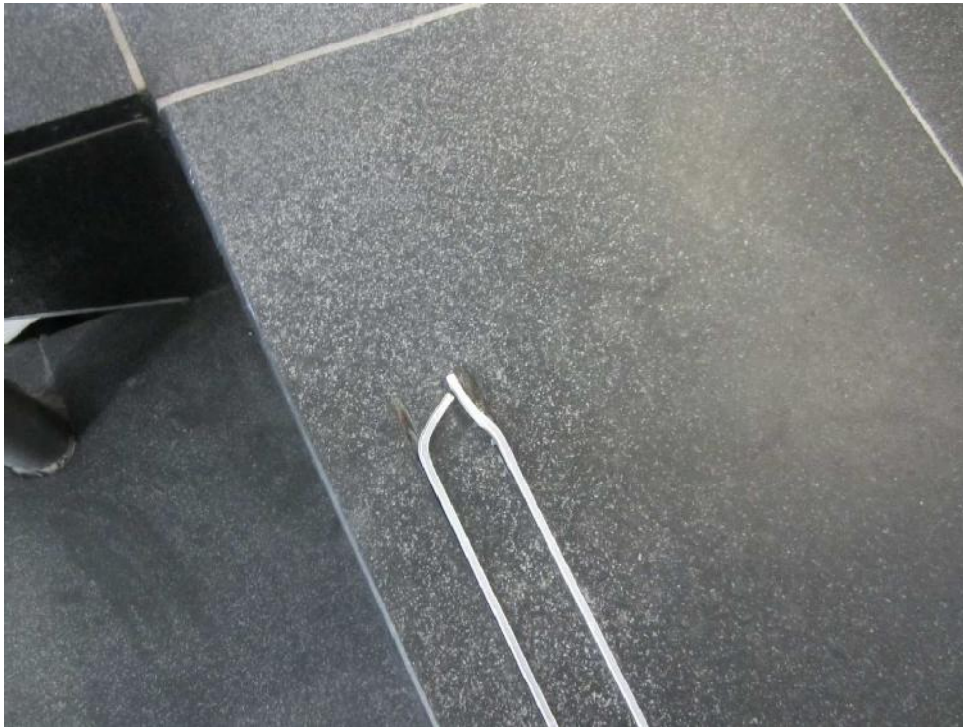
Photo 29: Metal tread strips to the main stair core are damaged.
