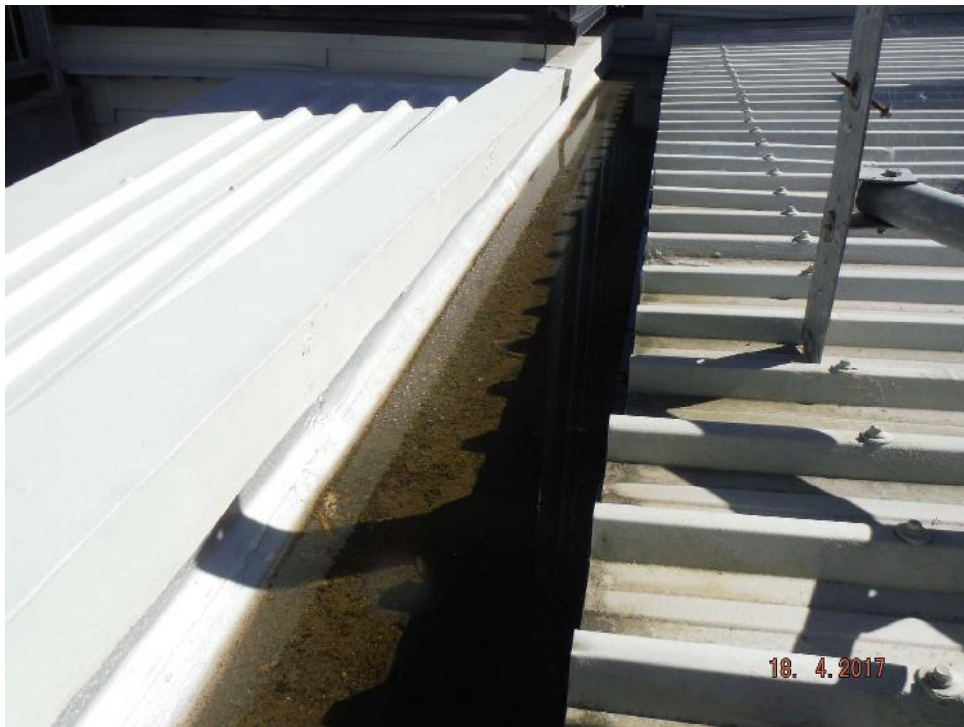
Photo 18: Ponding water to the membrane gutter.
