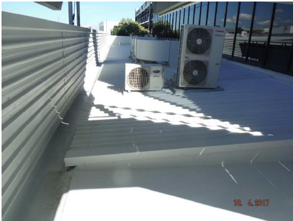
Photo 15: General view of the lower roof covered in trapezoidal metal sheets. A spray applied elastomeric coating has been used across the roof.
