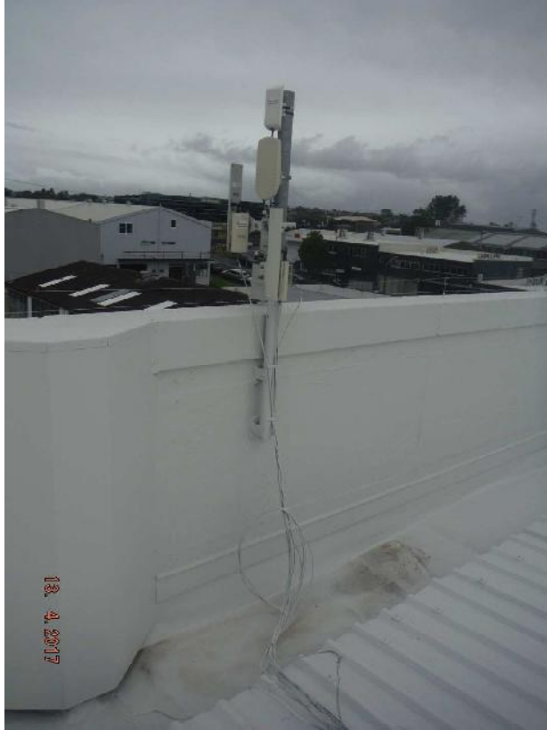
Photo 9: Cabling present to the roof. Any redundant roof items or cabling should be removed.
