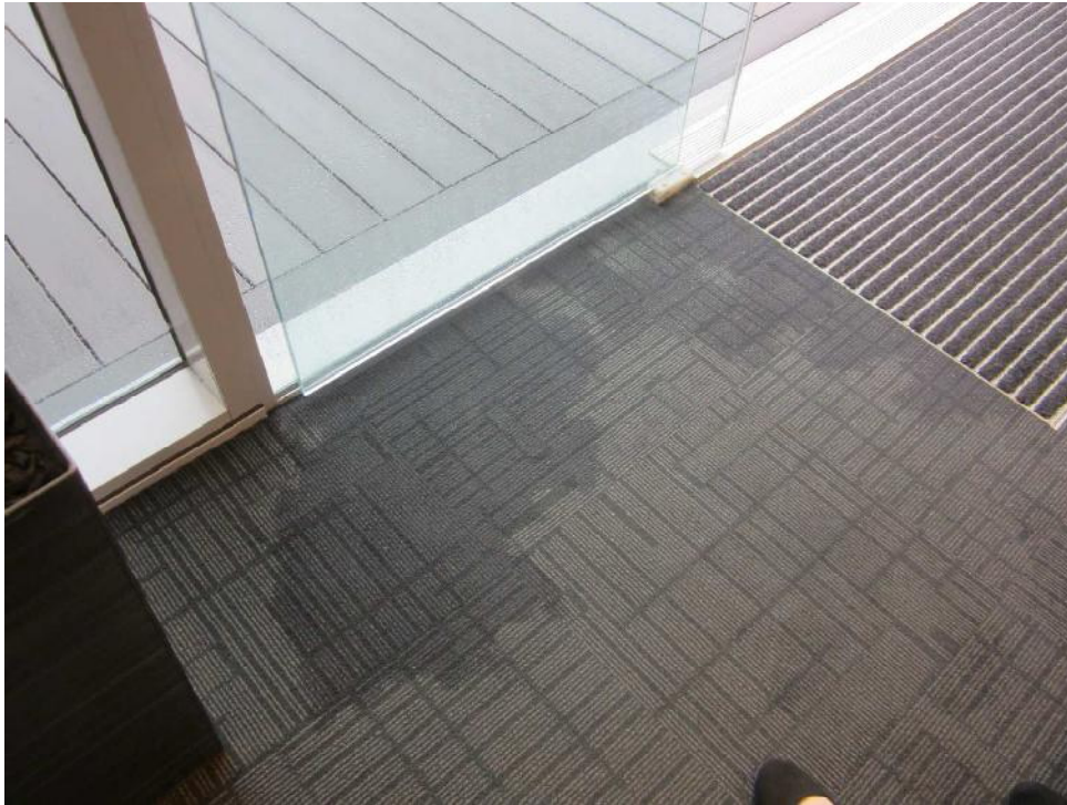
Photo 25: Water is entering the building adjacent to the radiology department doorway as a result of the poorly designed gutter.
