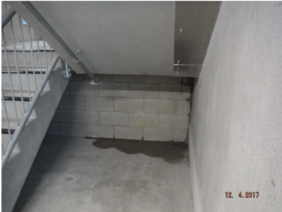
Photo 7: Water is entering the northern stair tower at ground level.
