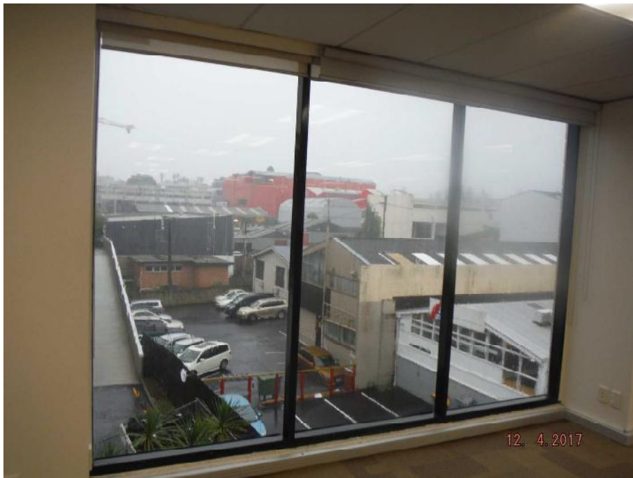
Photo 14: The specification of the full height glazing to the side and rear has not been confirmed. Non-compliant glass should be replaced with safety glass, or barriers should be installed.
