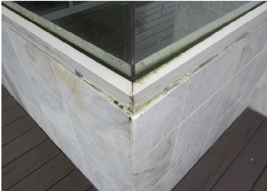
Photo 20: The age of the cladding system and the effects of UV degradation has resulted in hardened and shrunk seals. Sealant repairs have been applied to the stone veneer cladding joints, which are marked with algae and degrading.
