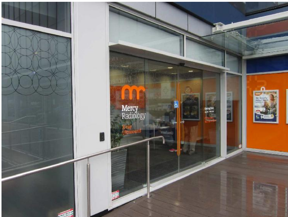
Photo 24: A gutter installed above the radiology department entrance door collects water off the canopy, which discharges against the glazed cladding.
