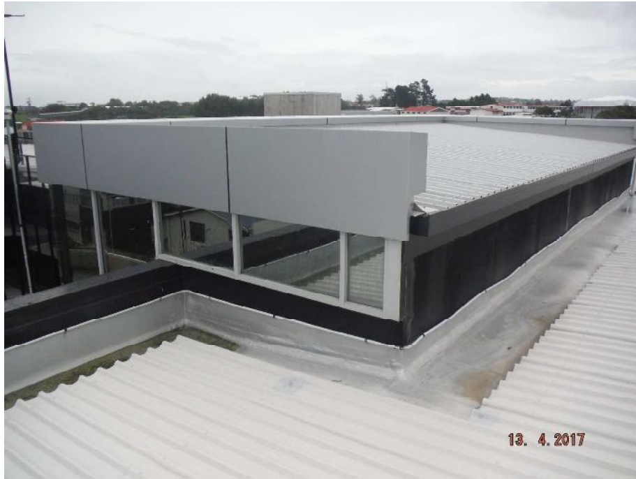
Photo 7: The metal roof covering over the main stair core appears is in good condition, although cyclone washers have not been installed to fixings. The junction between the parapet wall and window lacks adequate flashing cover and is high-risk from a weather-tightness perspective.
