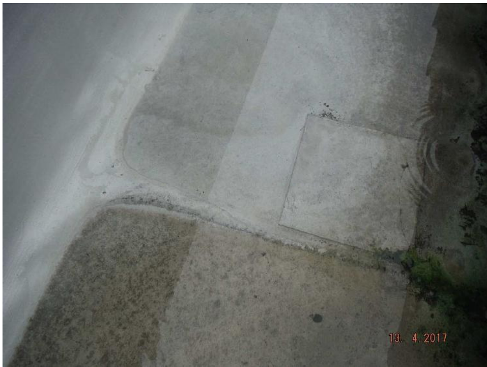
Photo 10: Ponding water noted to membrane gutters. Bubbling and evidence of previous patch repairs were also apparent.
