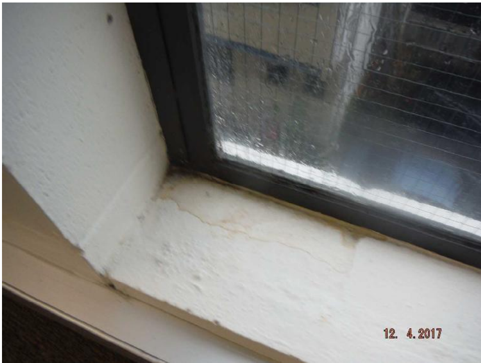
Photo 16: Water staining present to sills internally.
