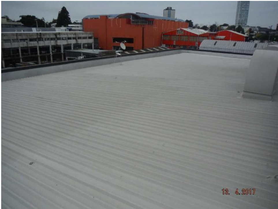
Photo 3: General view of the metal roof covering. The roof has been sprayed with an elastomeric coating to prolong its service life.
