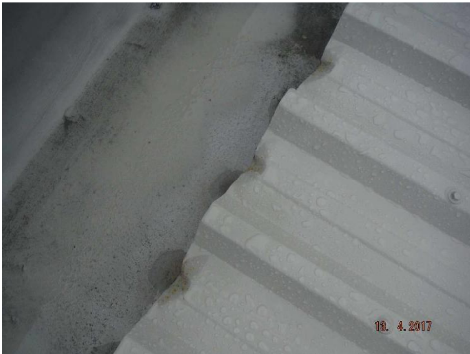
Photo 6: Surface corrosion to roof sheets is apparent through the coating.
