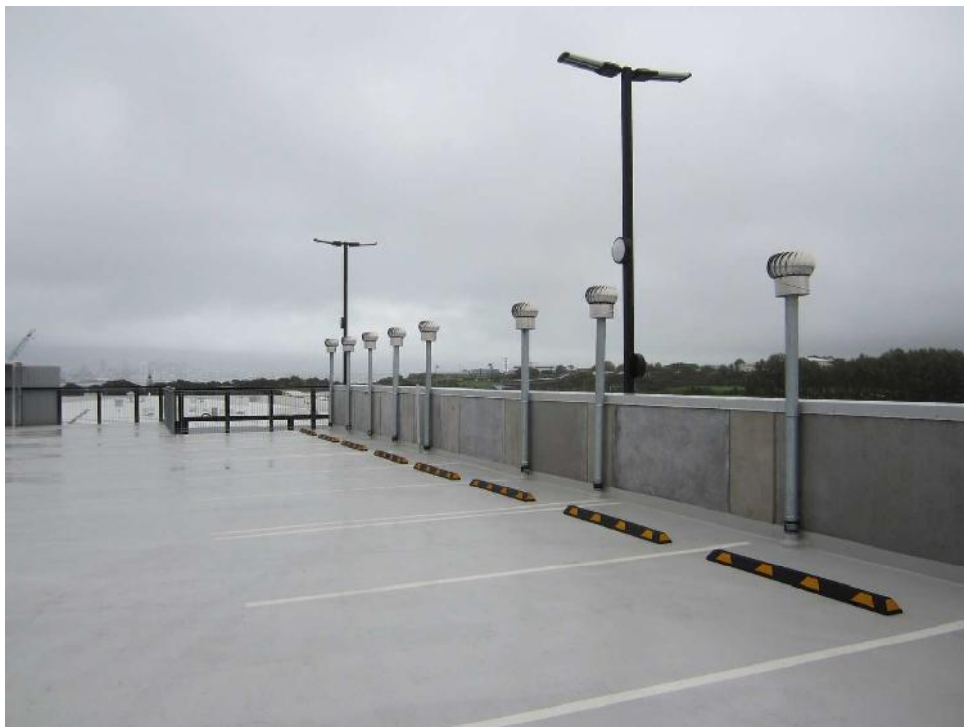
Photo 8: Wind driven cowls are installed at roof level as part of gas protection measures.
