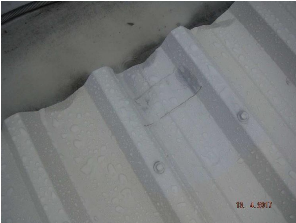
Photo 5: Flashing tape has been applied in numerous locations.
