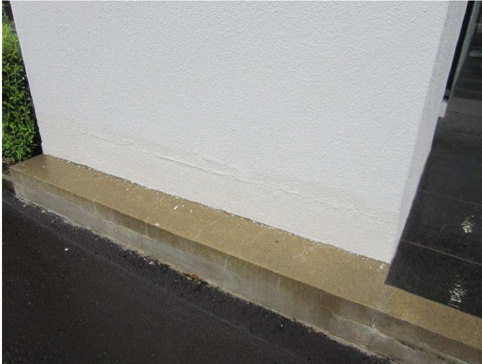
Photo 11: Previous damage to the render has been covered by the latest paint coat.
