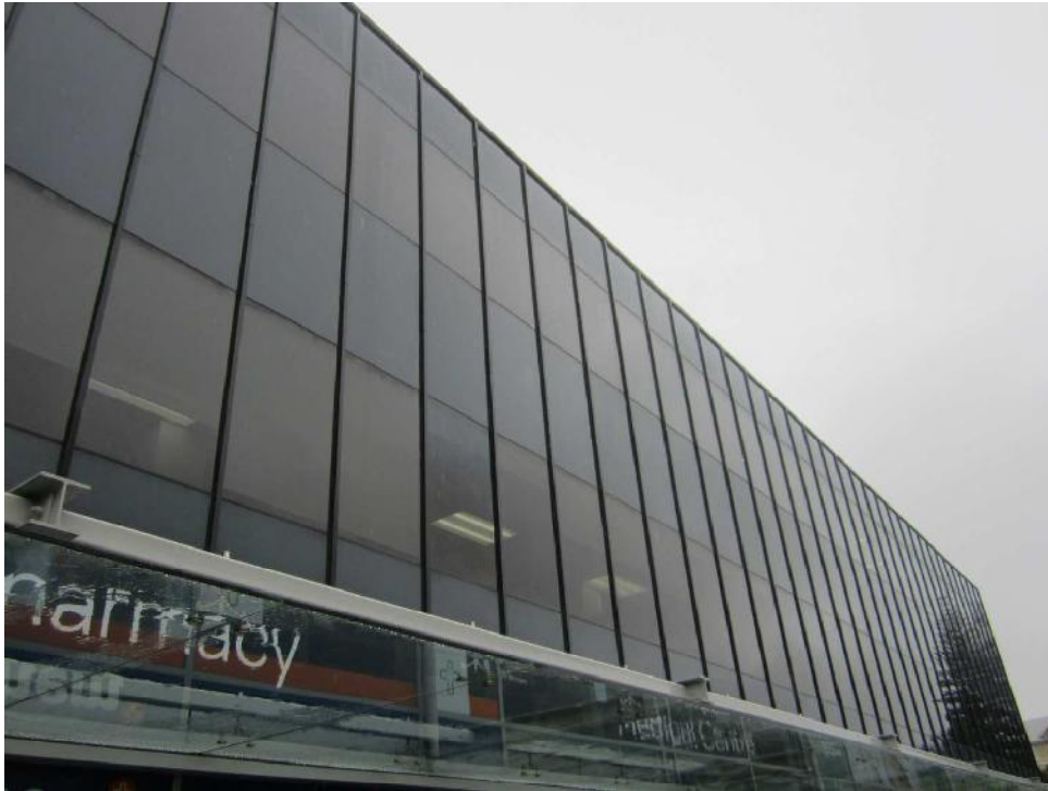
Photo 19: The cladding system to the upper level comprises glazed panels within aluminium mullion channels.
