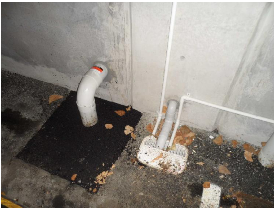
Photo 10: Service penetrations through a fire rated wall. The large penetration is labelled, but the smaller penetration is not and the fire stopping system is unknown.
