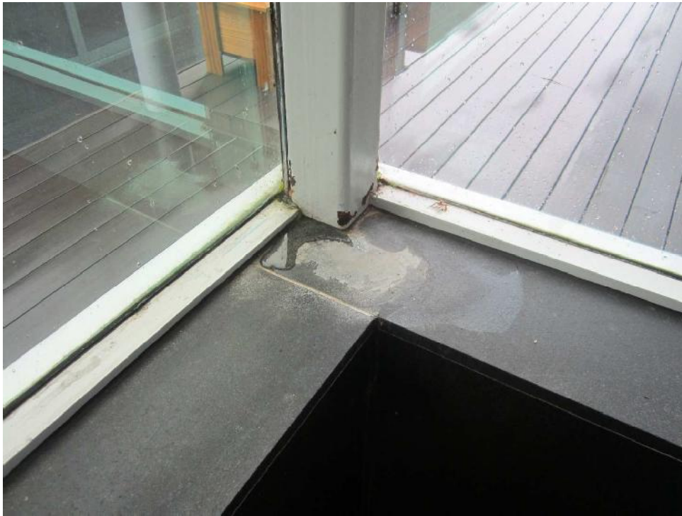
Photo 23: Water ingress noted within the main stair core. The water is likely entering at high level and tracking down.
