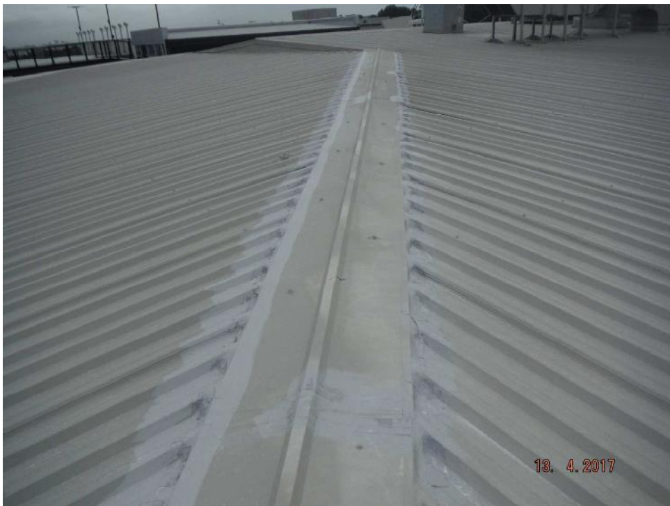
Photo 4: More recent repairs were also noted, such as brush applied elastomeric coatings to the hip capping.
