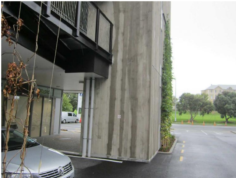
Photo 6: Water staining to the south stair tower.
