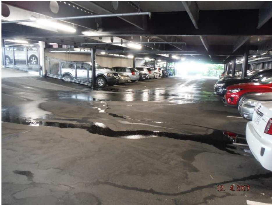
Photo 5: Water staining is present to the car park decks. Water management from the upper car park levels should be reviewed.
