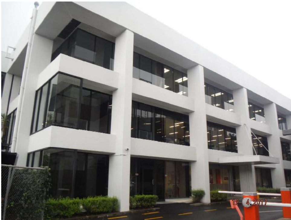
Photo 10: Elevations are finished with brush applied paint.
