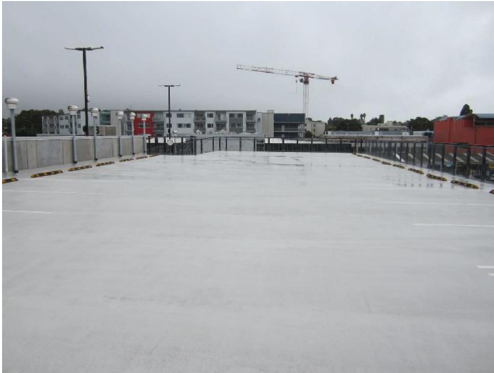
Photo 3: The upper deck to the carpark is coated with a flexible polyurethane waterproofing system.
