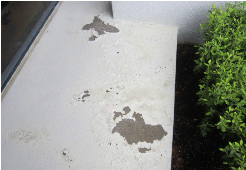
Photo 12: Window ledges are stained from water runoff and the paint surface is flaking. On going redecoration of the paint finish is required.
