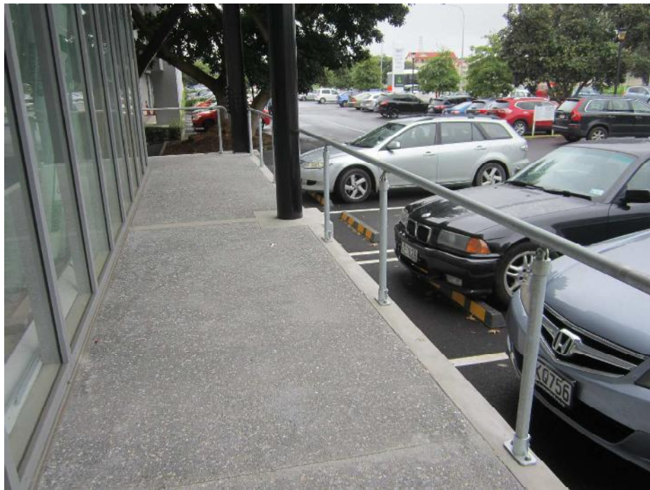
Photo 16: The handrail outside the building does not provide a barrier to children and should be reviewed. An upstand should also be installed to the edge of the ramp for disabled users.
