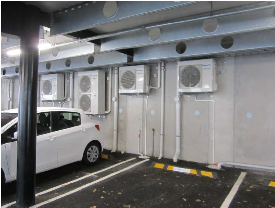
Photo 15: External condenser units located in the wall to the car park provide heating and cooling to internal areas.
