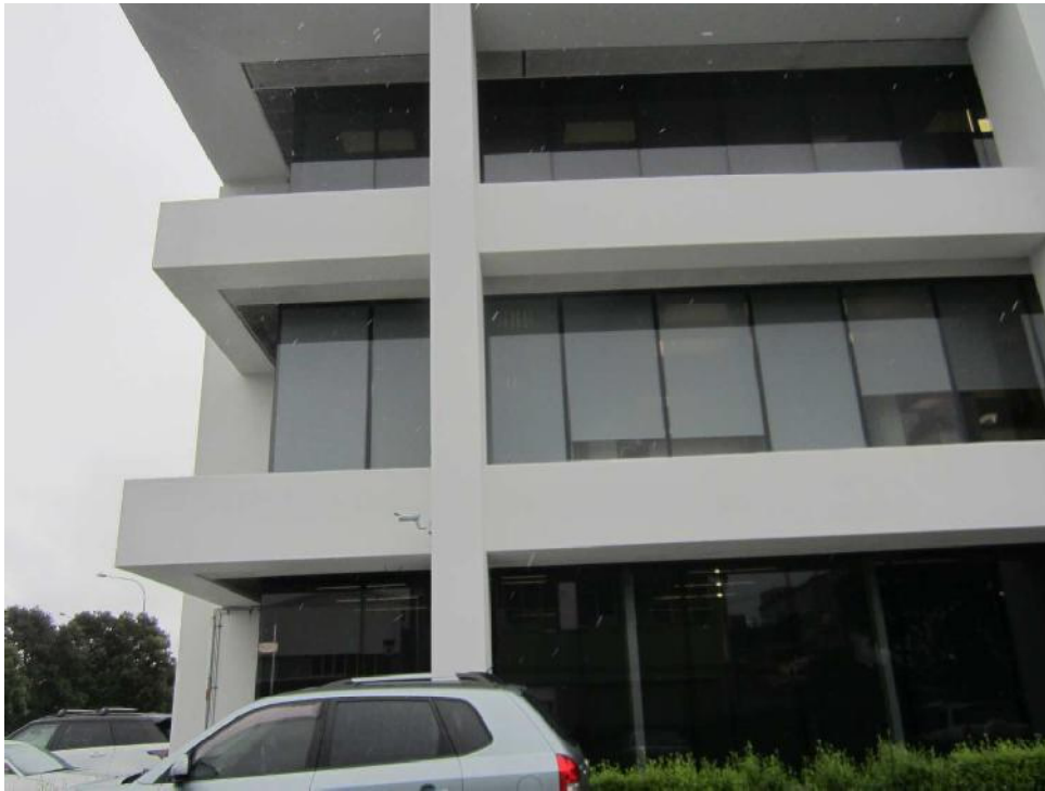
Photo 13: Aluminium framed windows installed throughout are recessed in to the elevation. Shrinkage and hardening of rubber seals was noted.
