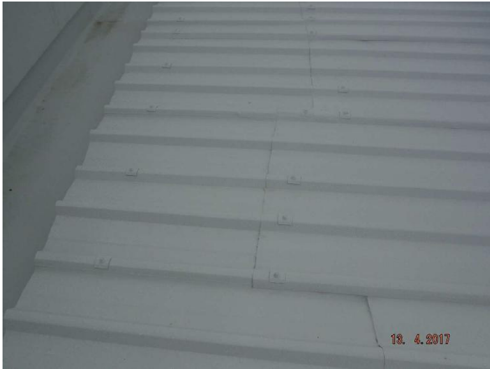
Photo 3: Evidence of previous patch repairs to roof sheets.
