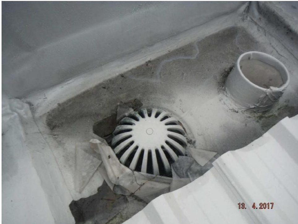
Photo 11: Gutter baskets and overflow pipes are installed throughout.
