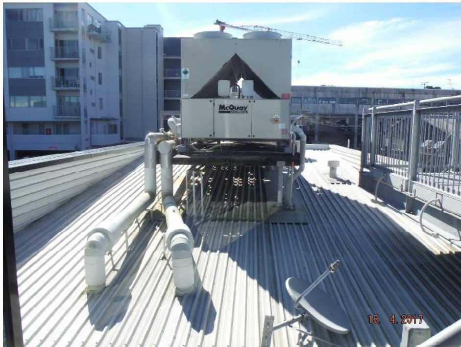
Photo 16: Air conditioning plant installed to the lower roof. Poorly detailed penetrations through roof sheets.
