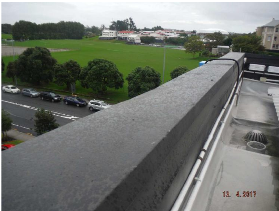
Photo 12: Parapet cappings include minimal falls and top fixings in some locations.
