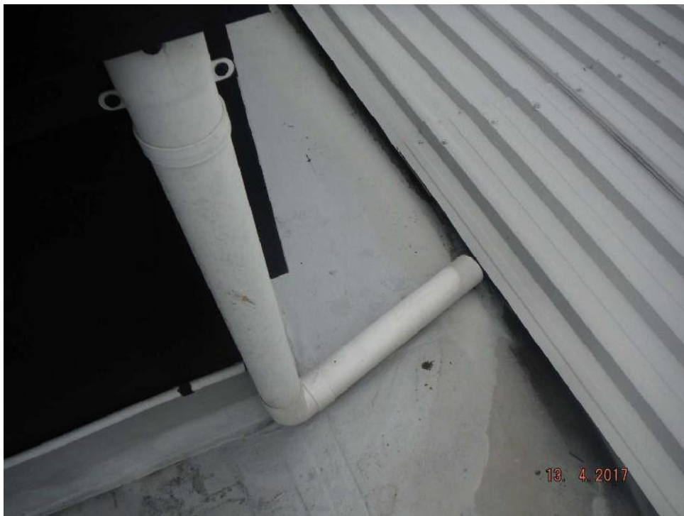
Photo 8: A downpipe from the stair core roof currently discharges against an unsealed roof edge; this should be reviewed.
