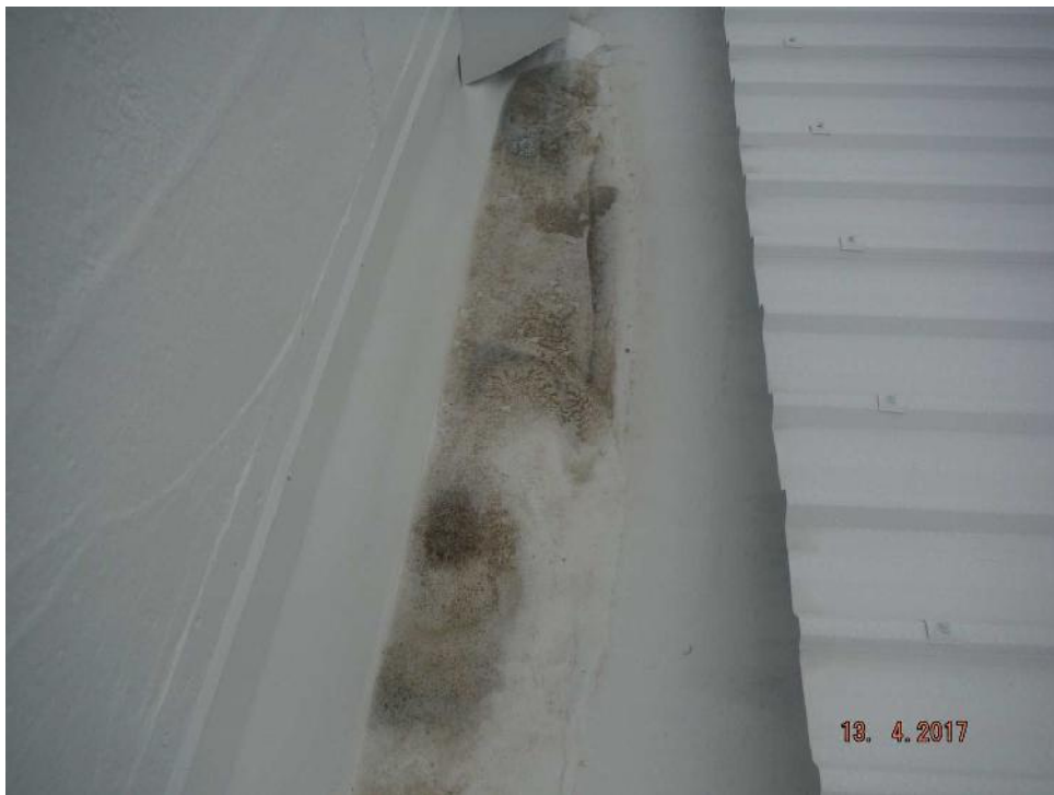
Photo 6: Ponding water evident to the membrane gutter. Bubbling and splits to the membrane were also noted.
