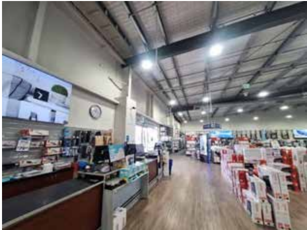
85. Example of the internal condition.
