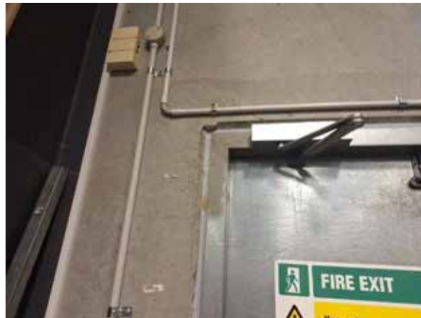
77. The internal sealant applied to the perimeter of the timber hinged doors were in a good condition.
