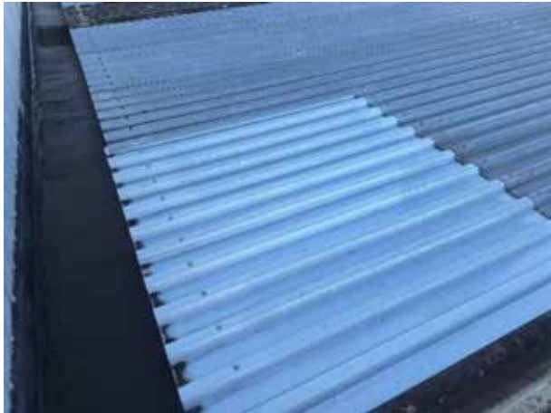
31. Localised targeted roof sheet replacement to the roof.
