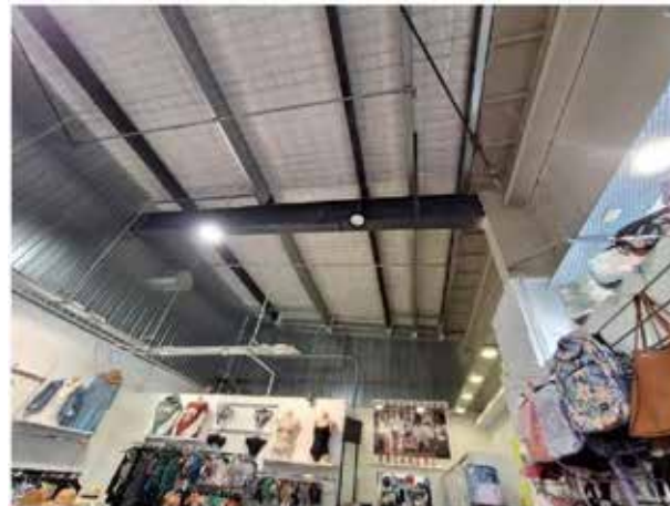
104. View of the underside of the roof (Chances Surf New Zealand).
