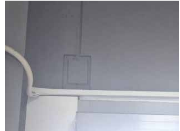
99. No corrosion was observed to the steel embedded plates. It is understood that this tenancy had been painted within the last year.
