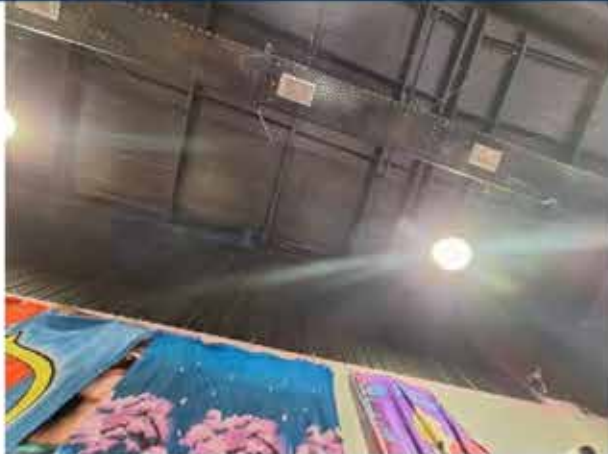
43. View of the underside of the roof (The Style Master).
