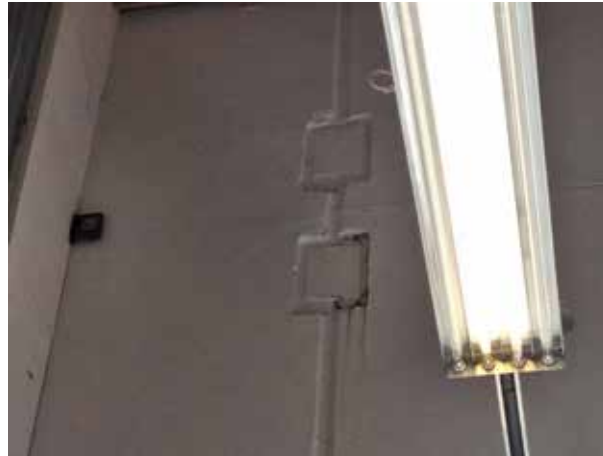
80. Widespread corrosion to the steel embedded plates of the concrete wall panels.
