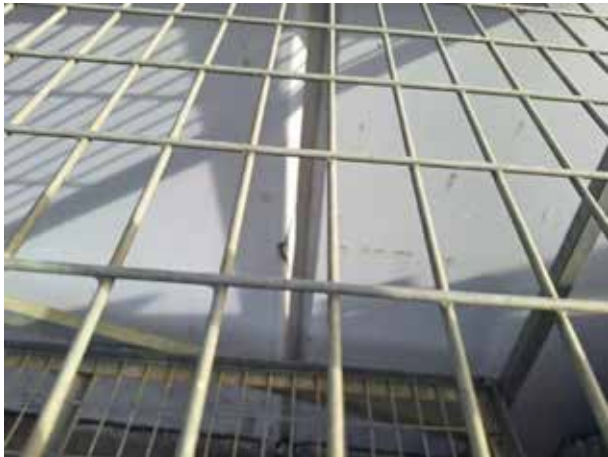
121. Sporadic areas of abrasions, deterioration and spalling to the concrete wall panels.
