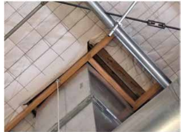
48. View of the underside of the roof (The Baby Factory).
