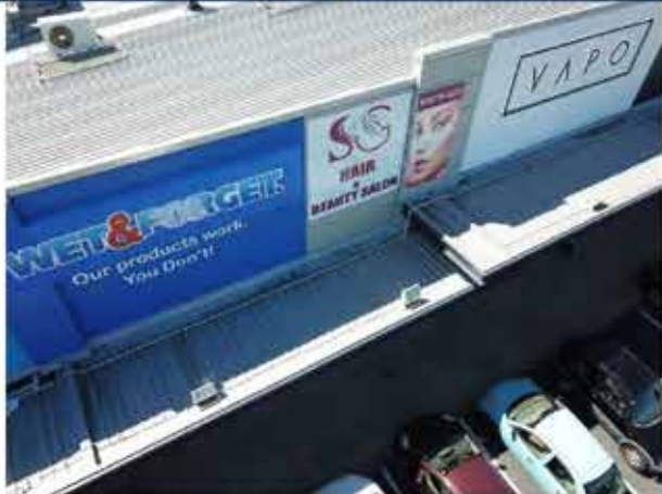
127. View of the upper side of the canopy roofs.
