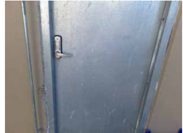
39. Sporadic areas of minor abrasion and deterioration to the concrete wall panels.
