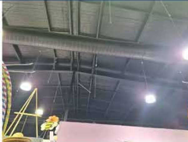
44. View of the underside of the roof (The Style Master).
