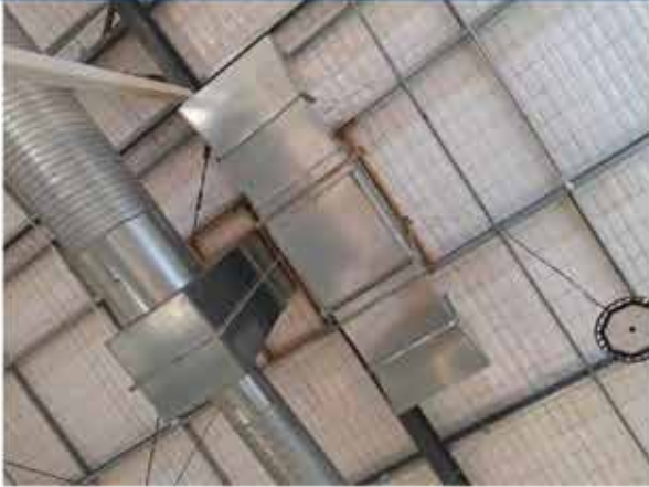
112. View of the underside of the roof (Carpet Court).
