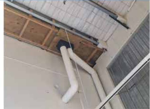
51. View of the underside of the roof (The Baby Factory).
