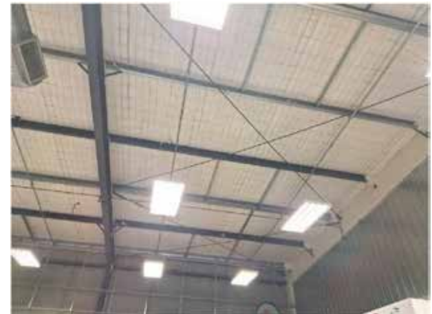
54. View of the underside of the roof (Tool Shed).
