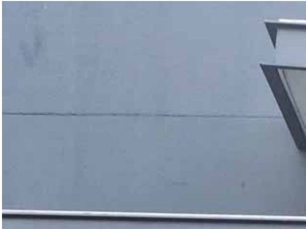
25. Localised former signage markings to the upper-level horizontal signage.
