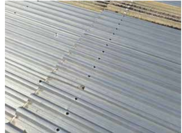
57. Sporadic areas of sealant applied to the profiled metal roof sheets.
