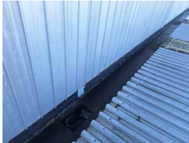
71. Sporadic areas of targeted repair sealing works to the joints of the synthetic membrane sheets.
