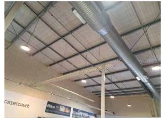
111. View of the underside of the roof (Carpet Court).
