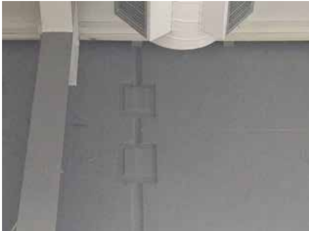
100. No corrosion was observed to the steel embedded plates. It is understood that this tenancy had been painted within the last year.
