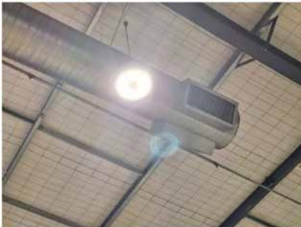
58. View of the underside of the roof (Bed Bath and Beyond).
