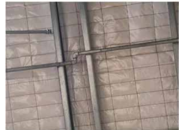
126. Underside of the roof with minor wrinkling to the underlay and a service pipe.
