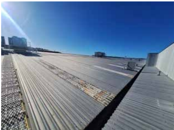
4. The profiled metal roof sheets were typically in good condition.
