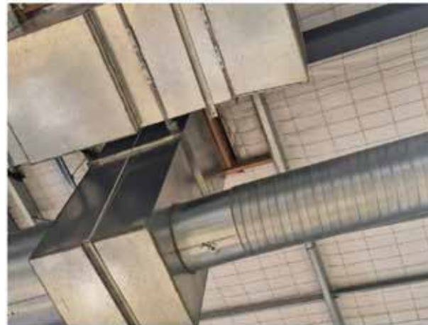
59. View of the underside of the roof (Bed Bath and Beyond).
