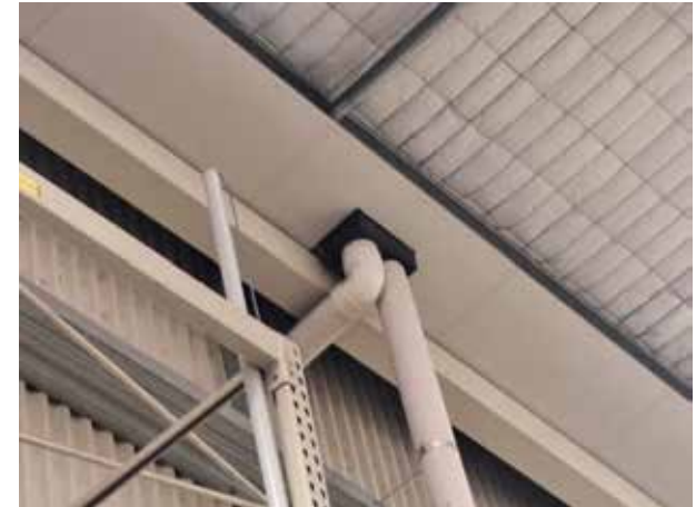
183. The underside of the internal gutters were in a good condition with no leaks observed at the time of the inspection.
