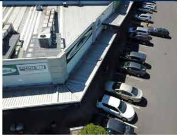
80. View of the upper side of the canopy roofs.
