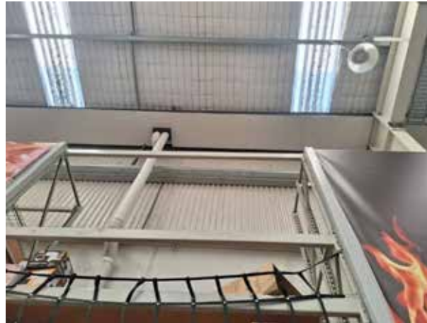
182. The underside of the internal gutters were in a good condition with no leaks observed at the time of the inspection.
