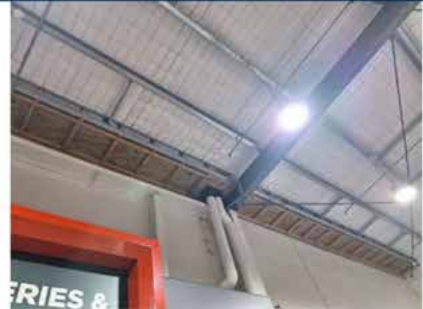
39. View of the underside of the roof (RepcO).
