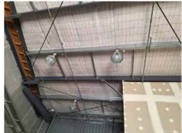
30. View of the underside of the roof (Fruit World).
