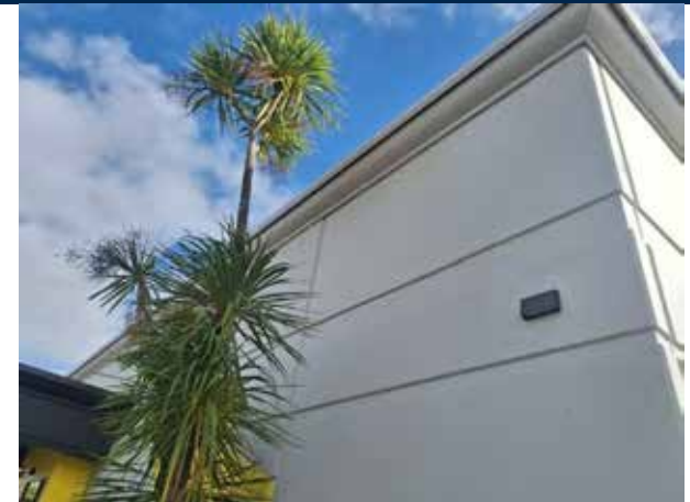
3. The paint condition was generally in a good condition to the elevations.
