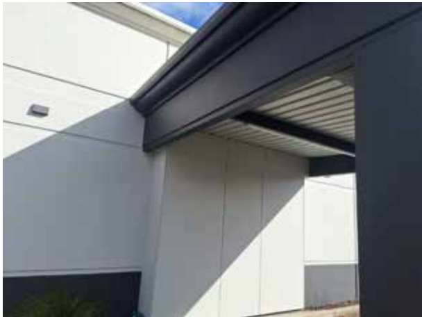
4. The paint condition was generally in a good condition to the elevations.
