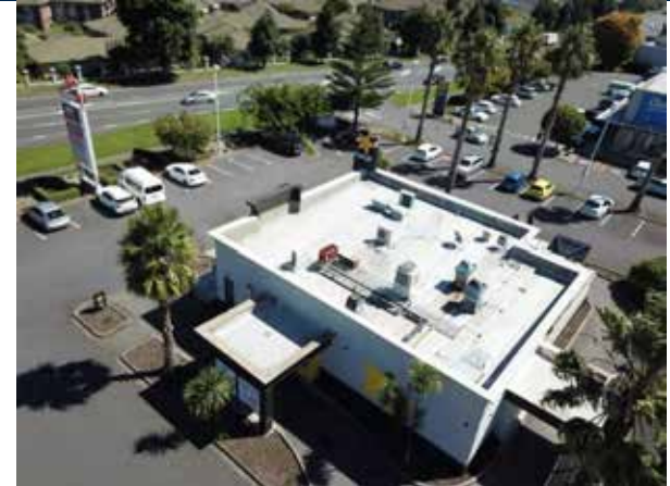
132. View of the roofs.
