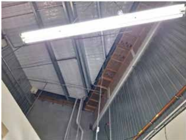
34. View of the underside of the roof (Liquorland).
