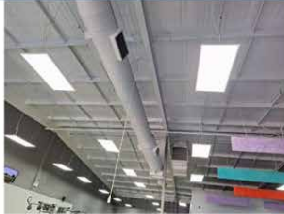
113. View of the underside of the roof (Anytime Fitness).
