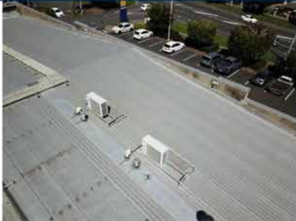
100. Extensive sealant applied on the fit-over flashings and around the EPDM boot flashings.
