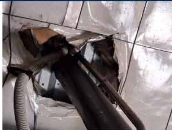
56. Services penetration through the profiled metal roof sheets.
