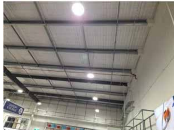
119. View of the underside of the roof.
