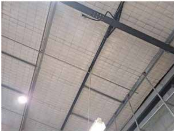
64. View of the underside of the roof (Harvey Norman).
