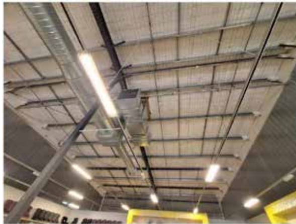
47. View of the underside of the roof (The Baby Factory).
