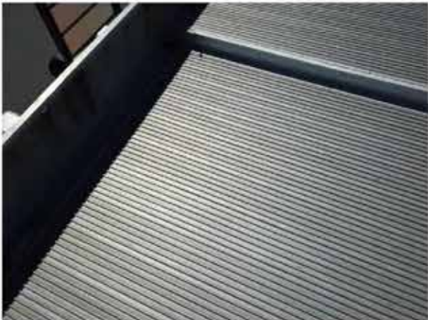
22. Profiled metal roof sheets.
