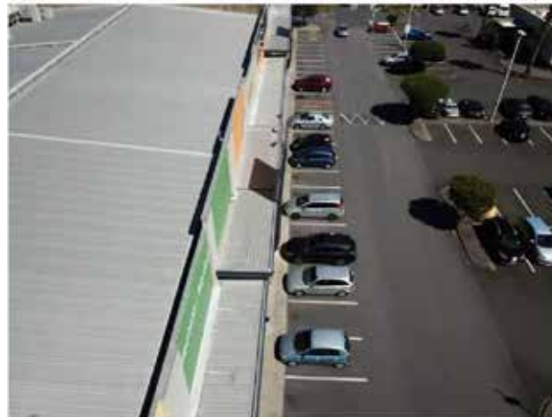
77. View of the upper side of the canopy roofs.
