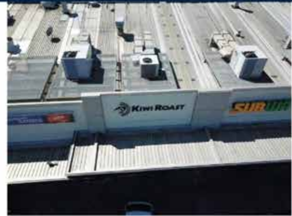
81. View of the upper side of the canopy roofs.
