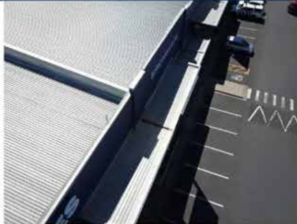
128. View of the upper side of the canopy roofs.
