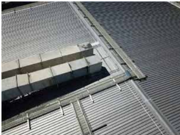
85. Extensive sealant applied to the kerb penetrations and fit-over flashings.
