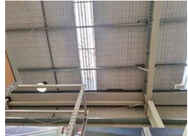
180. The underside of the roof was in a good condition with no leaks observed at the time of the inspection.
