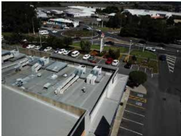
76. View of the upper side of the canopy roofs.
