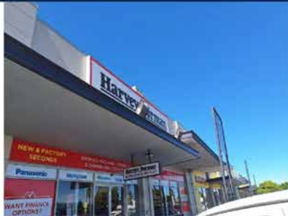
74. View of the underside of the canopy roofs.
