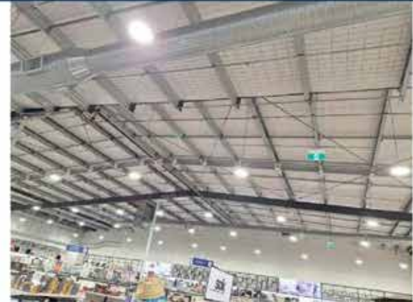
108. View of the underside of the roof (Briscoes).
