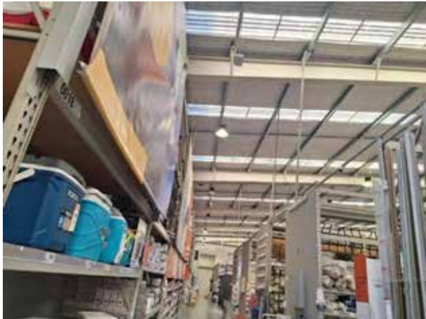
181. The underside of the roof was in a good condition with no leaks observed at the time of the inspection.
