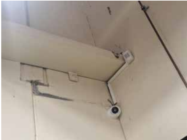
91. Sporadic areas of previous repairs to the control joints and steel embedded plates within the concrete wall panels.
