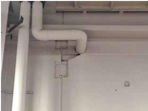
88. Widespread corrosion to the steel embedded plates of the concrete wall panels.
