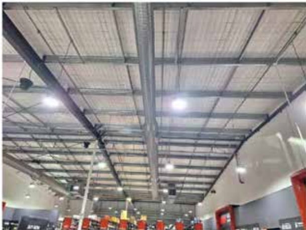
40. View of the underside of the roof (RepcO).
