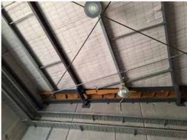
28. View of the underside of the roof (Fruit World).
