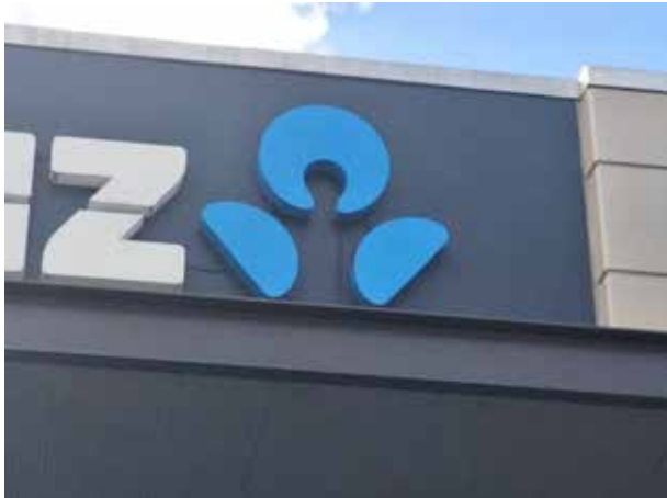
52. Localised discolouration to the upper-level horizontal concrete wall panels at the southern elevation.
