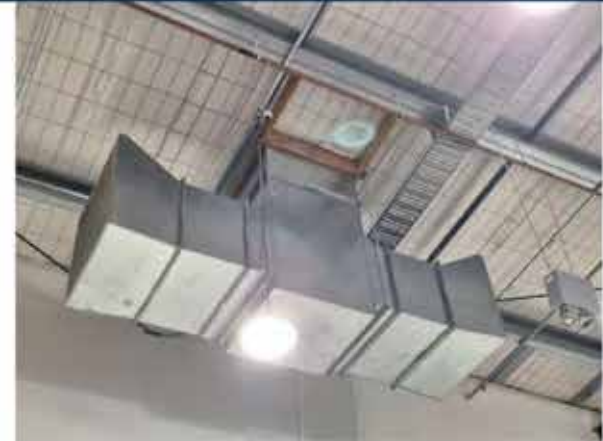
117. Localised staining on the timber framing for the large penetration.
