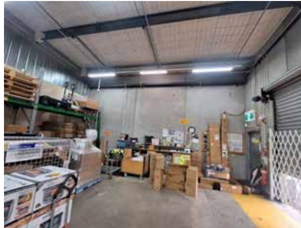
92. Example of the internal condition.
