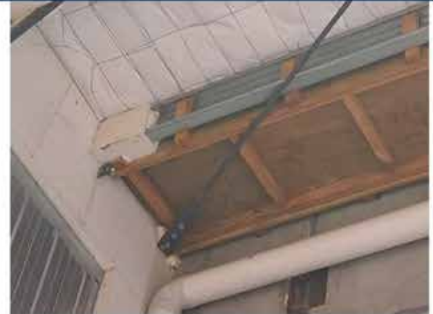
69. No evidence of staining to the plywood substrate (Tool Shed).
