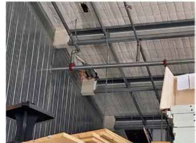
36. View of the underside of the roof (Liquorland).
