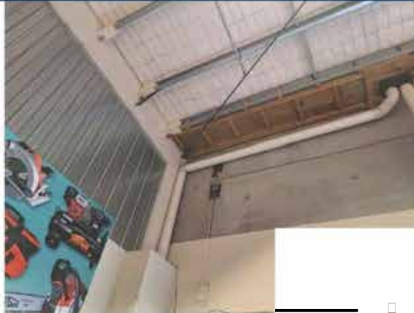
68. View of the underside of the roof (Tool Shed).
