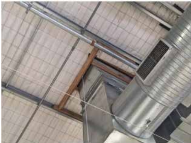
52. View of the underside of the roof (Harvey Norman).
