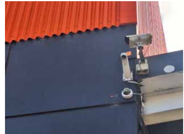
96. Localised redundant fixing centres to the concrete wall panels.
