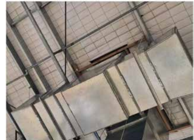
60. View of the underside of the roof (Bed Bath and Beyond).
