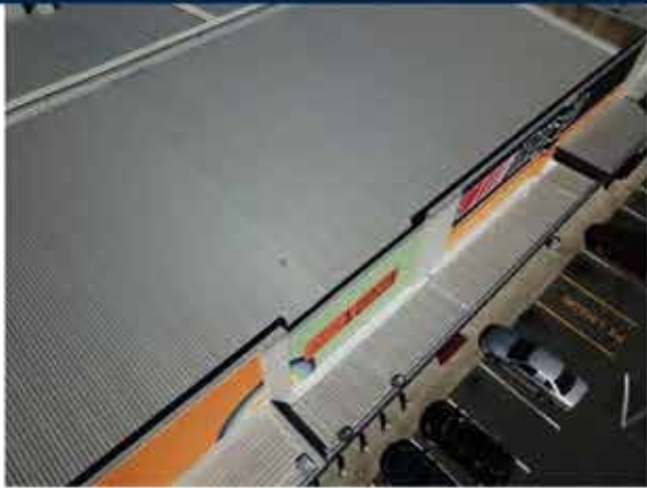
79. View of the upper side of the canopy roofs.
