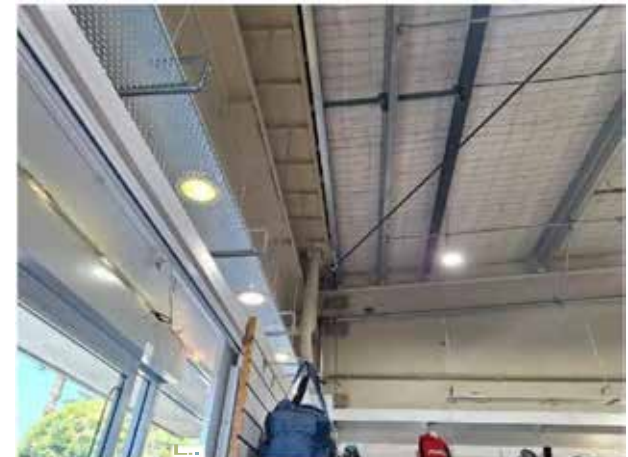
105. View of the underside of the roof (Chances Surf New Zealand).
