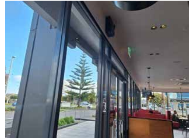
21. Internal view of the elevations.
