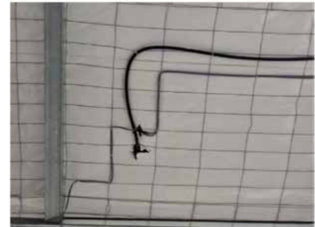
120. A cable penetration was observed within this area.
