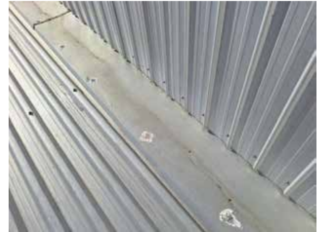
60. Widespread sealant applied to the fixings of the apron flashings.
