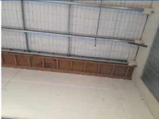
67. View of the underside of the roof (Harvey Norman).
