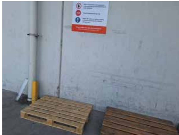
101. Sporadic areas of abrasions, deterioration and spalling to the concrete wall panels.
