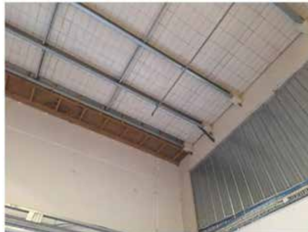
53. View of the underside of the roof (Harvey Norman).
