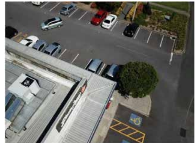
78. View of the upper side of the canopy roofs.
