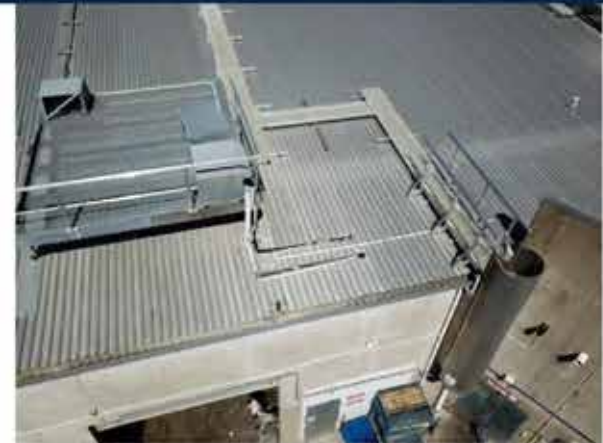
57. Sealant applied around the services penetrations.
