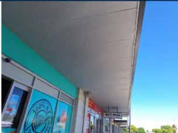
73. View of the underside of the canopy roofs.
