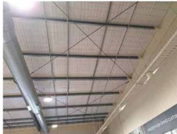
110. View of the underside of the roof (Carpet Court).
