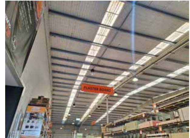
192. The underside of the roof was in a good condition with no leaks observed at the time of the inspection.
