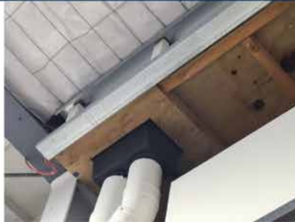
116. View of the internal gutters within Briscoes.
