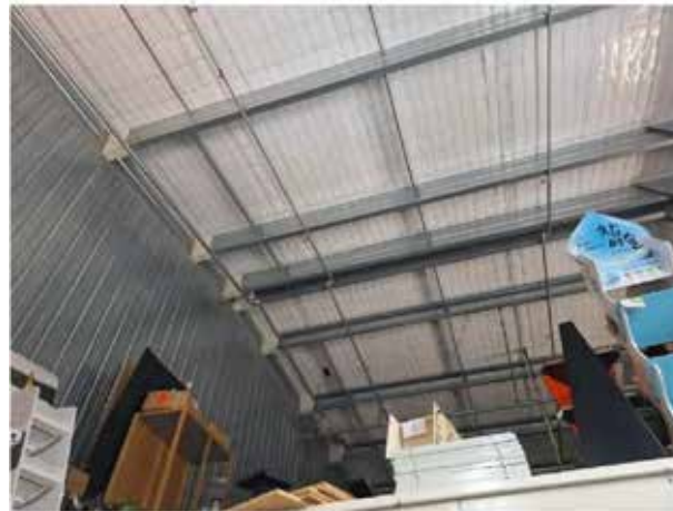
35. View of the underside of the roof (Liquorland).
