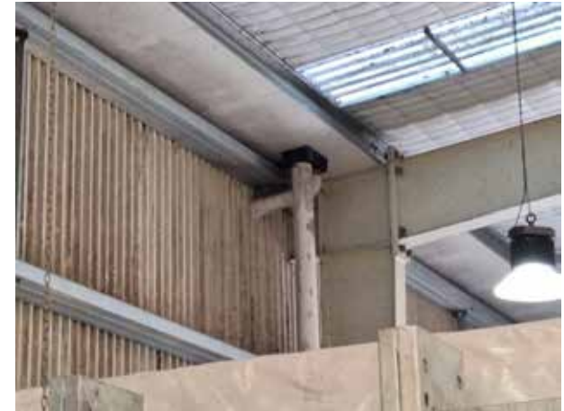
207. The underside of the rainwater goods were in a good condition with no leaks observed at the time of the inspection.
