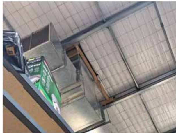
41. View of the underside of the roof (RepcO).
