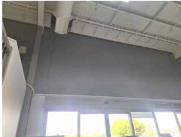
98. Example of the internal condition.
