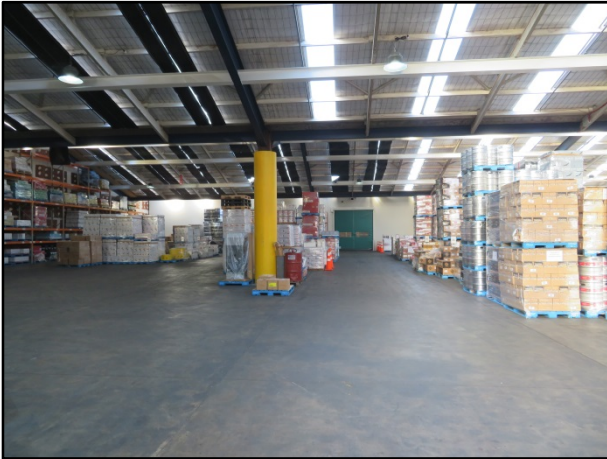
Toll covered yard area
