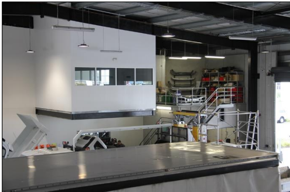
Training room cantilever
