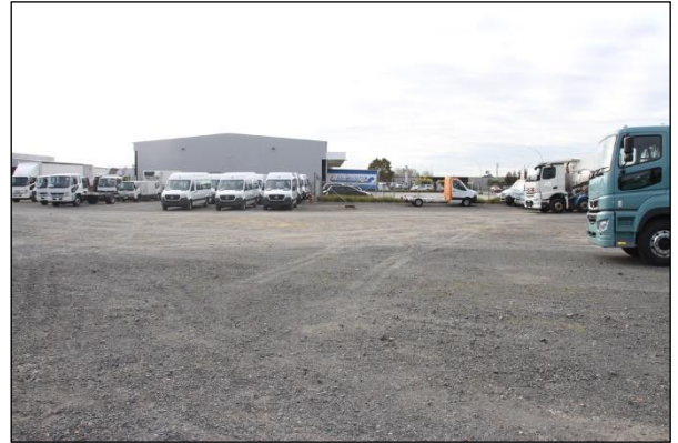
Western elevation and metalled yard
