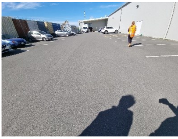
12. Typical view of hardstandings to north carpark area.
