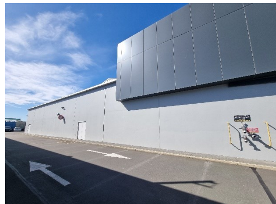
6. West elevation of Block A.
