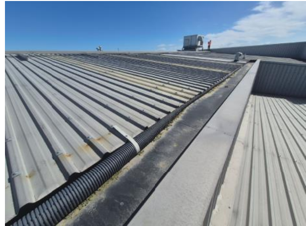
H16 – Block C roof internal gutter with drainage coil
