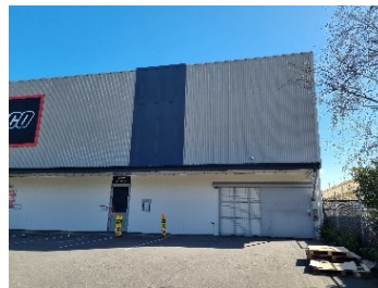
46. Block C - Aluminium composite panels utilised to localised areas.
