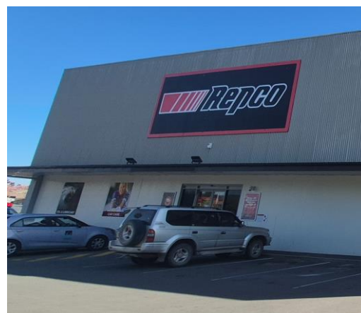
E12 – External signage LED flood uplighting
