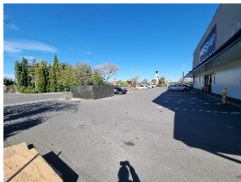
9. Typical view of hardstandings to east carpark area.
