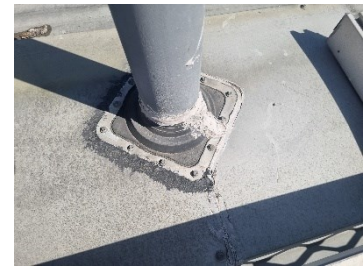
41. Block C - Sealant applied around boot flashings to service penetrations.
