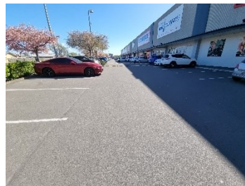
10. Typical view of hardstandings to south carpark area.
