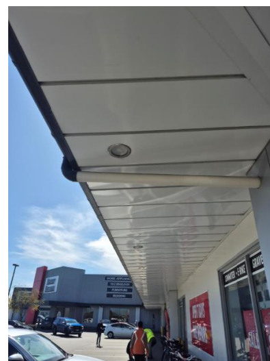
H12 –External hosetap without vacuum breaker
