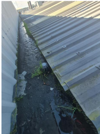
H15 – Typical Block C internal gutter
