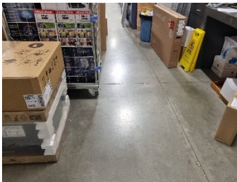
72. Block A - Concrete floor to northern warehouse extension.
