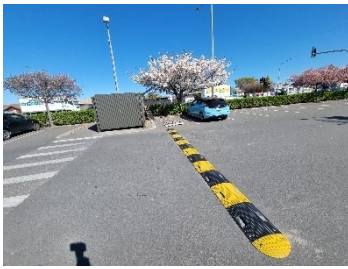
15. Speed humps to carpark.
