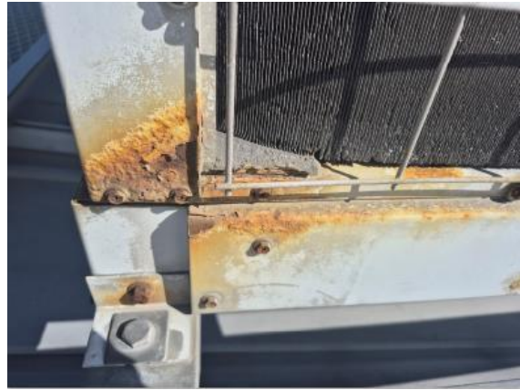
M2 – Block C PAC unit with moderate corrosion on chassis rails
