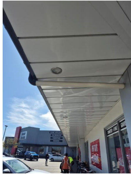
H14– Typical downpipe from eave gutter
