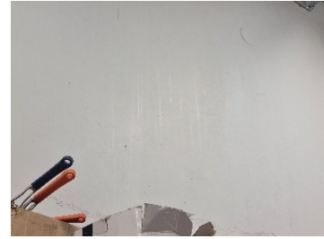
65. Block A - Moisture staining along interior face of east wall to warehouse corridor.
