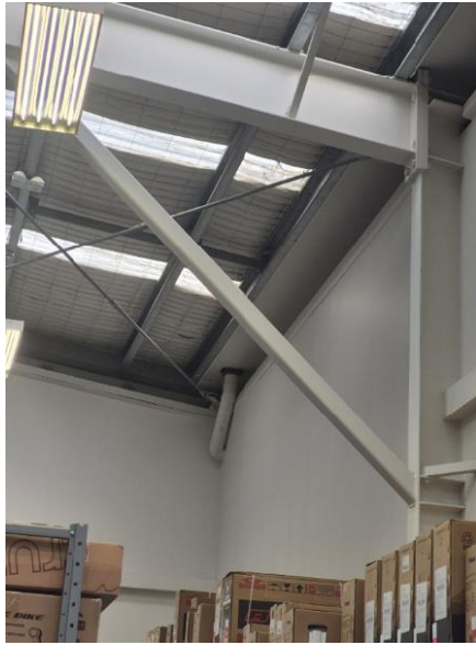
H13 – Block C Internal gutter downpipe
