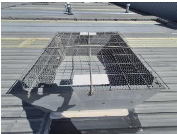
M5 – Smoke extract complete with bird/vermin mesh
