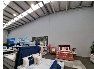
71. Block C - Typical view of intertenancy wall (Photograph, retail unit 9).
