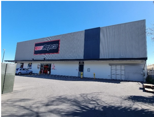
1. East elevation of Block C.
