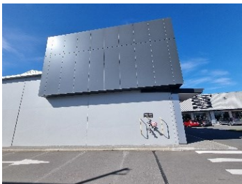
45. Block A - Aluminium composite panels utilised to localised areas.
