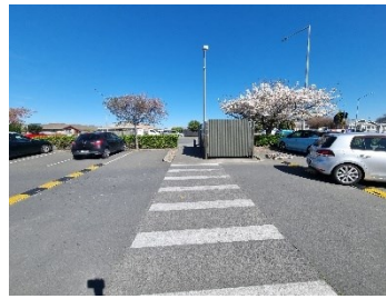
16. Bin structures to south and east of carparks. Bin structure to south obstructed view of and from crossing.
