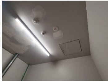
55. Block A - No access to roof from ceiling hatch to west exit.
