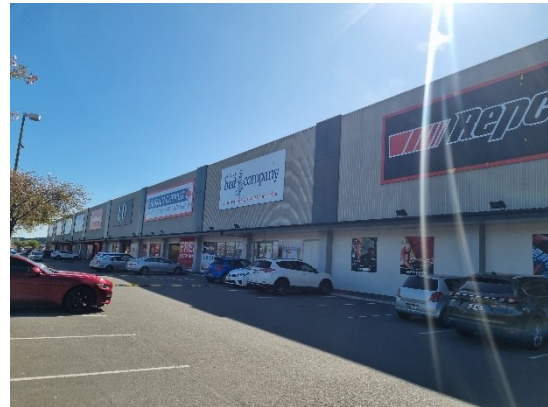
2. South elevation of Block C.
