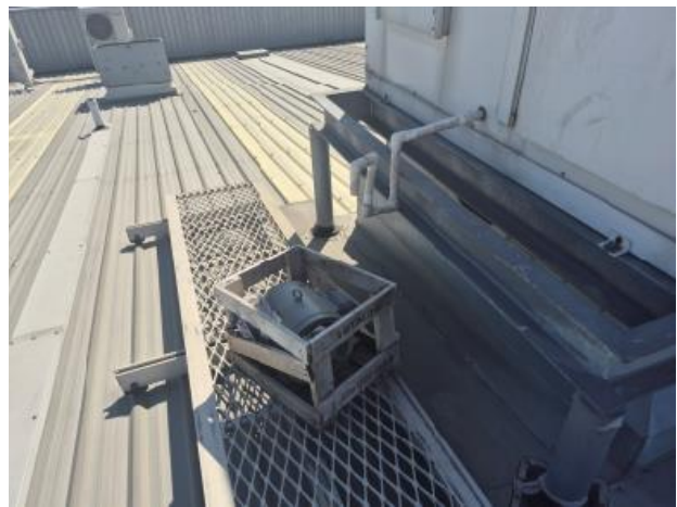
M2 – Block C PAC unit with moderate corrosion on chassis rails
