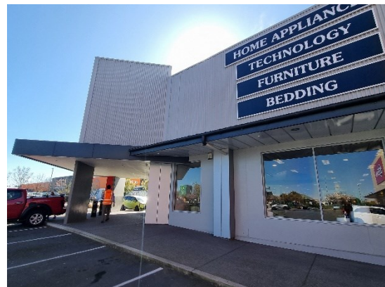
4. South elevation of Block B.
