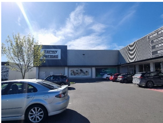
5. West elevation of Block B and south elevation of Block A.
