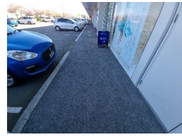
14. Concrete paving slabs to walkways beneath storefront canopies.
