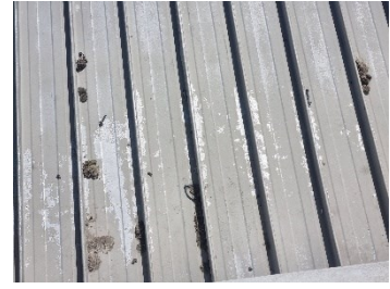
29. Block B - Surface finish of roof cladding delaminating exposing bare metal underneath.
