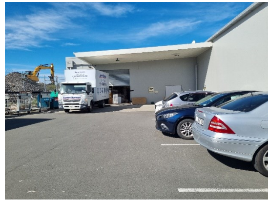
8. Partial west elevation of Block A.
