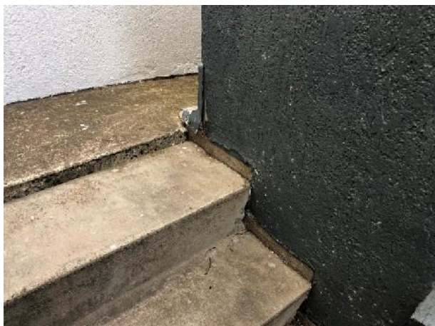
Minor subsidence to concrete path
