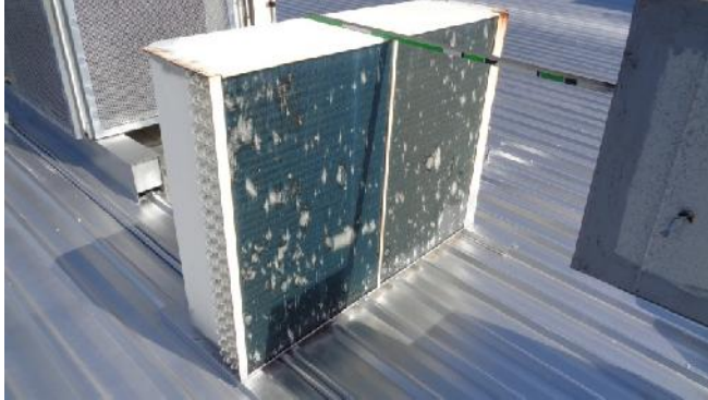
Hail damaged condenser
