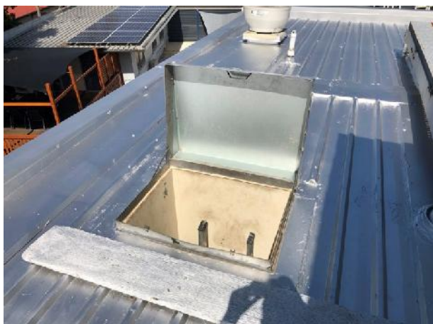
Building A1/3 Unsafe roof access
