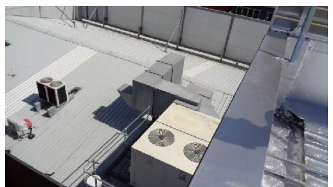
Roof mounted condensers
