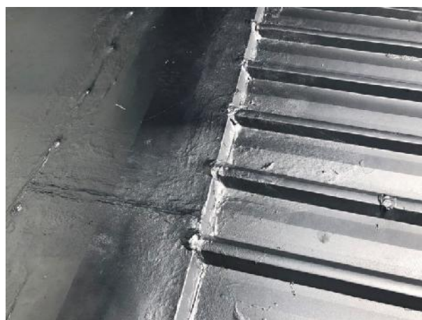
Building A1/3 Capping scribe break sealed
