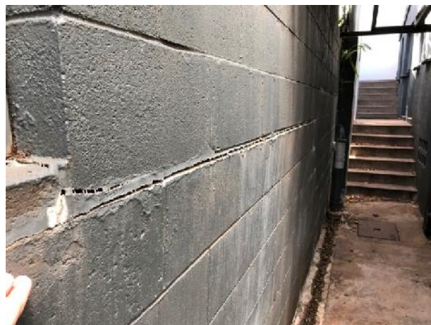
Bulge to retaining wall
