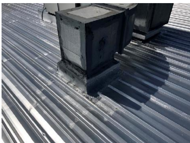
Building A1/3 Inadequate flashings
