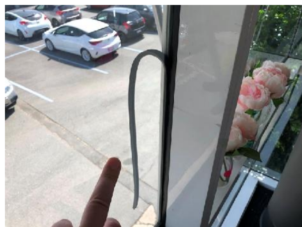
Typical window gasket dislodgement
