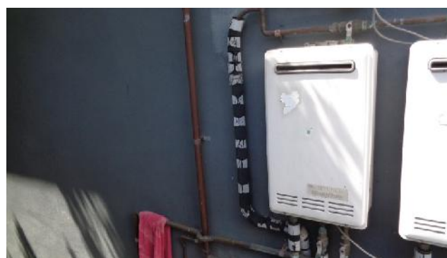
Gas fired water heaters
