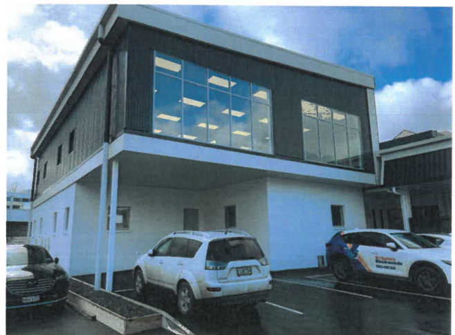
New Building Addition
