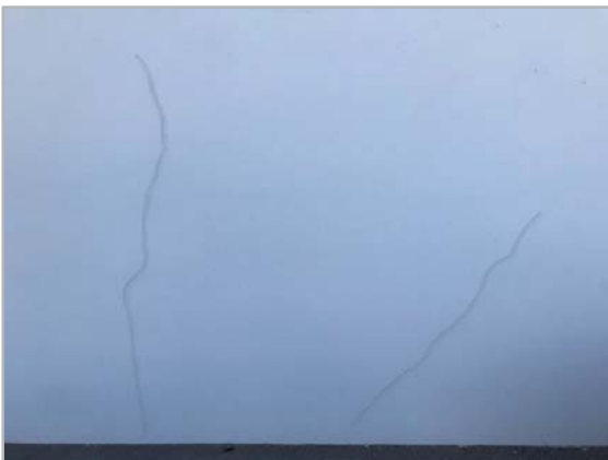
29. Repaired Cracking to Pre-Cast Panels, Unit 12
