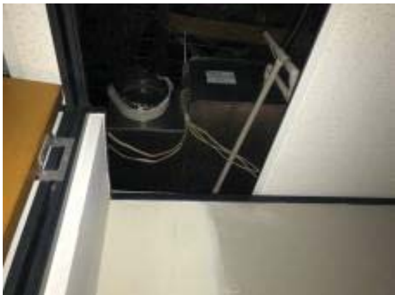
3. Vacancy ceiling works
