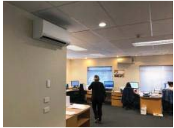
20. Wall hung split air conditioning (typical)
