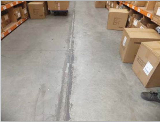
31. Typical Unpainted Floor Slab, Unit 4
