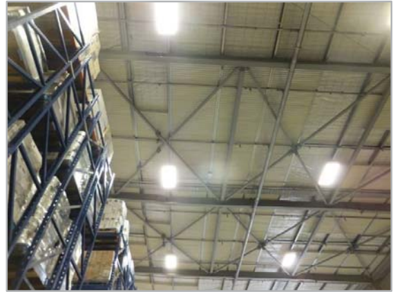
20. Diagonal Bracing Used to Unit 9 Roof Structure
