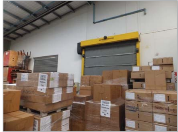
38. Roller Shutter Openings in Inter-Tenancy Wall, Unit 15
