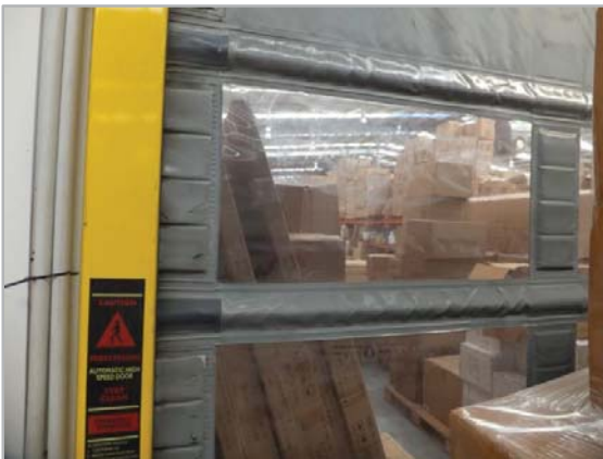
39. Poor Security in Inter-Tenancy Wall, Unit 15
