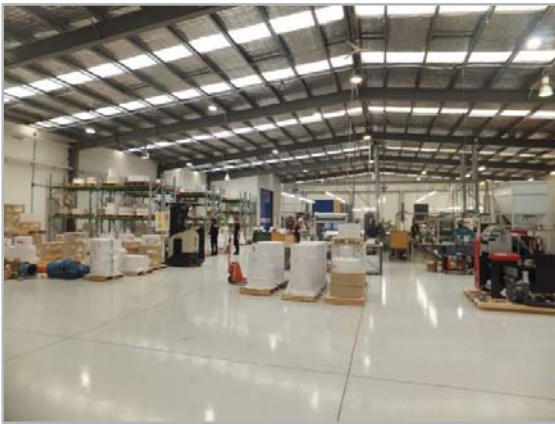
33. Painted Floor Slab, Unit 6
