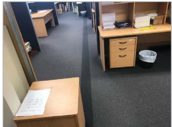
40. Evidence of Post-Earthquake Repairs, Unit 17
