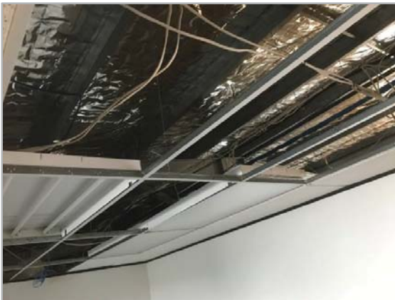
23. Underside of Roof, Unit 10A Chapmans Road
