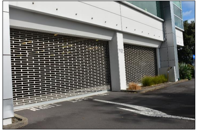
Secure carpark entrance
