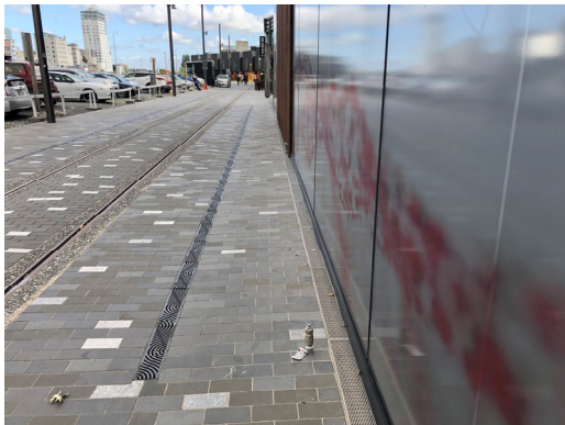
1.27. General view of tram lines and side road
