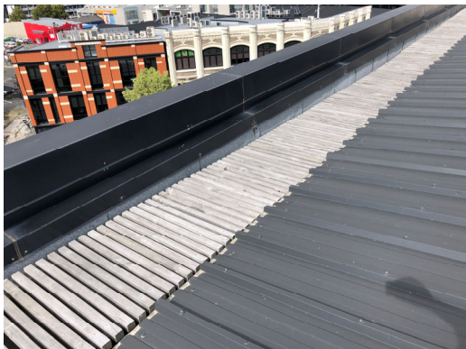
1.5. Timber walking boards to perimeter of roof
