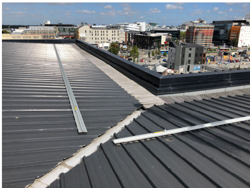
1.3. General view of roof areas
