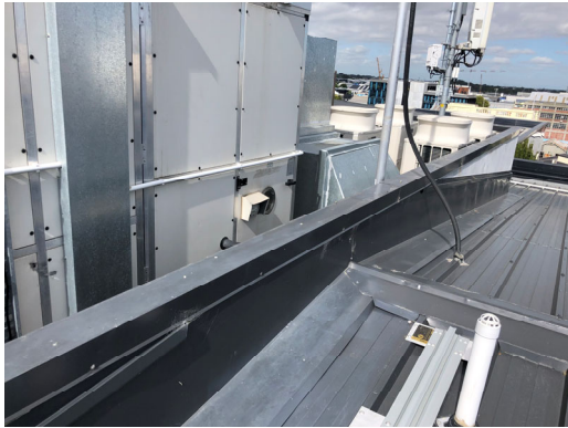
1.7. View of cap flashing
