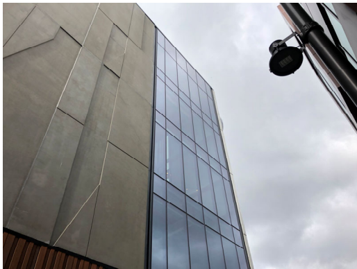
1.41. General view of north elevation
