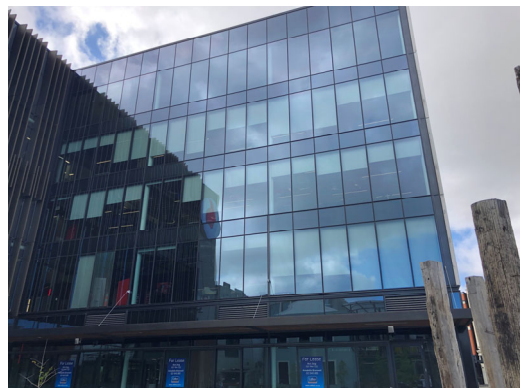
1.12. View of external elevations
