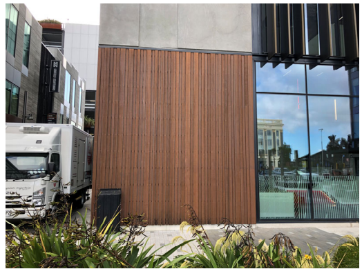
1.16. Vertical stained timber cladding
