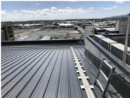
1.9. View of harness anchor points
