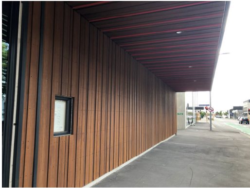
1.31. View of timber cladding to south elevation
