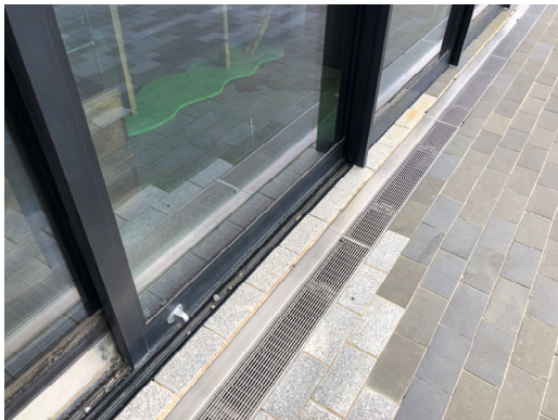
1.21. View of sliding door track and Aco Drain
