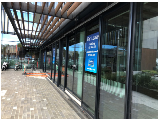
1.23. View of office frontage
