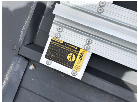
1.10. Harness anchor point information plate
