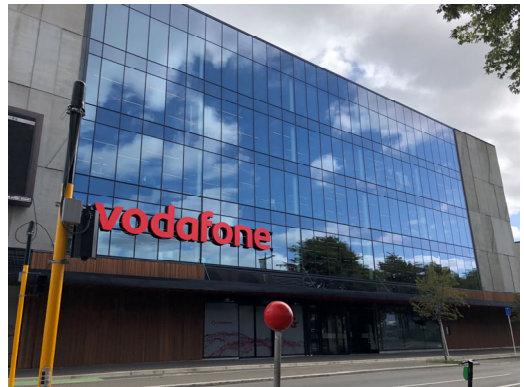
1.28. General view of south facing elevation
