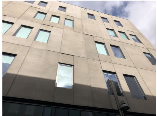
1.38. Precast concrete elevations
