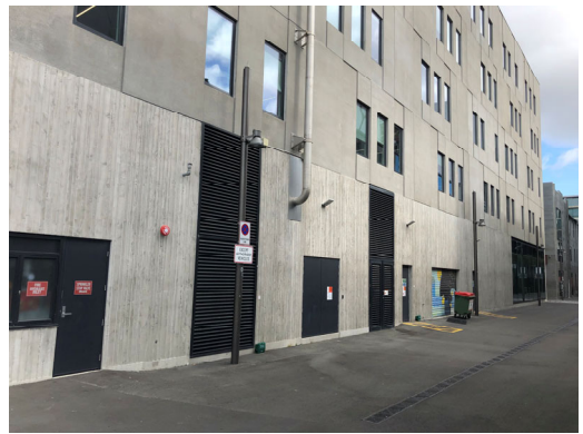
1.34. View of east elevation
