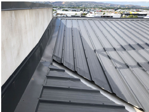
1.4. General view of roof areas
