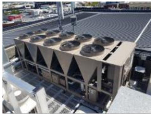
M16 – AHU VRF Outdoor Unit on Roof
