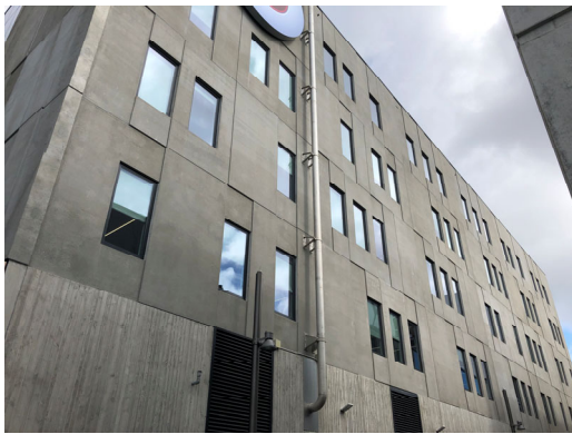
1.33. View of east elevation
