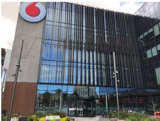
1.11. View of external elevations
