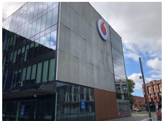
1.24. Concrete panels to external elevation
