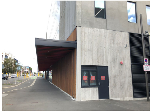
1.32. South east corner of building
