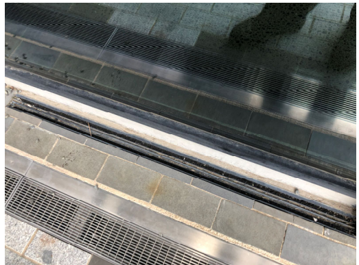
1.22. View of sliding door track and Aco Drain
