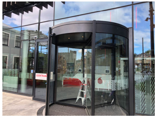
1.18. Main entrance under repair
