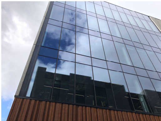
1.39. General view of glazed curtain walling
