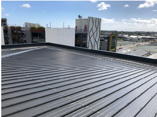
1.2. General view of roof areas
