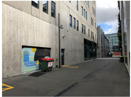
1.36. General view of east access road
