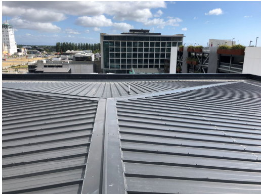
1.1. General view of roof areas
