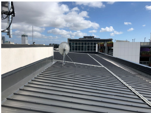
1.6. General view of roof areas
