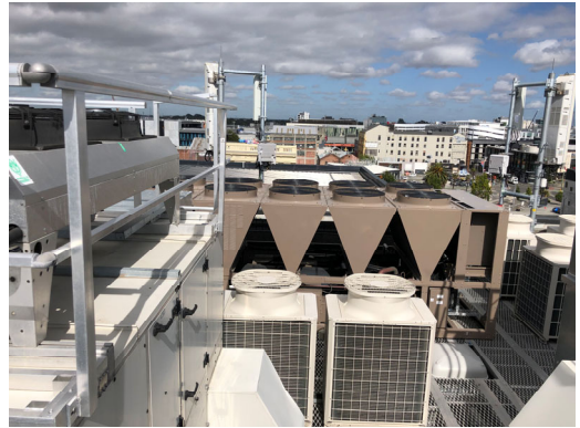
1.8. General view of plant areas
