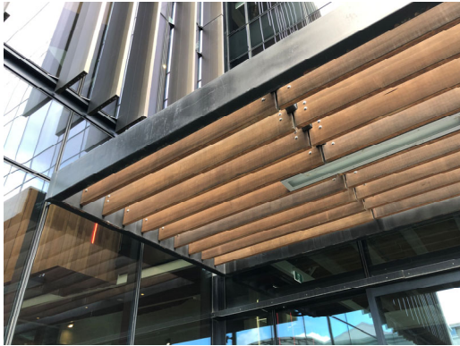
1.19. View of canopy
