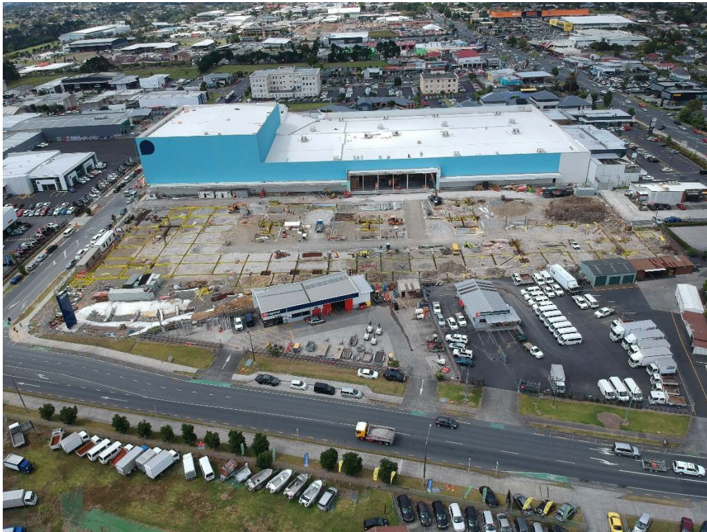
Photos of nearly completed "Nido" building at 156-160 Central Park Drive (January 2020)
