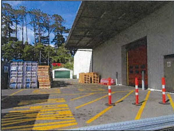
Good Health – Warehouse Canopy & Yard
