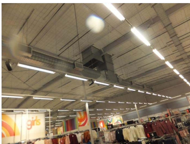
Supply and return air penetrations, K-Mart tenancy
