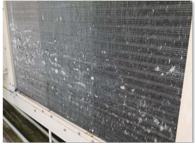
Deteriorated coils to packaged unit.
