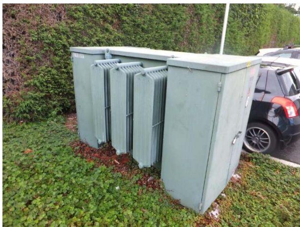
1,000 kVA substation
