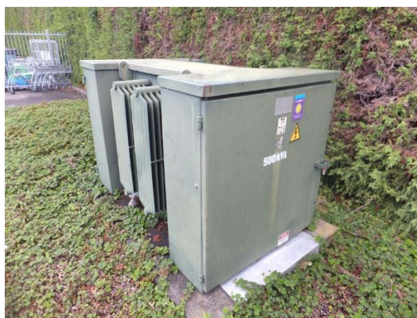
500kVA substation
