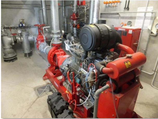
Sprinkler pumpset, Block E
