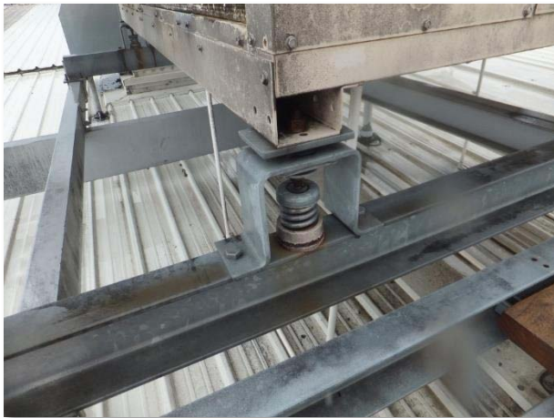
Packaged unit - soiled cabinets and corroded mounts
