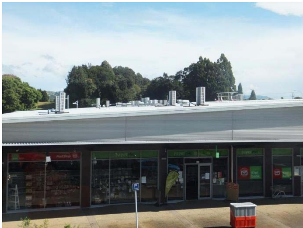
Typical split system units on Block C
