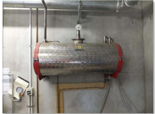
Diesel tank, Block E
