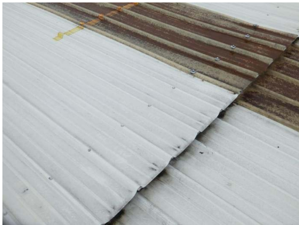
Rooflights to supermarket roof
