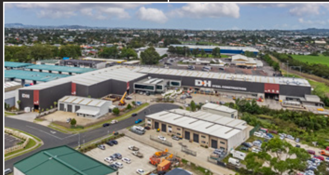
12 BRICK STREET, HENDERSON
