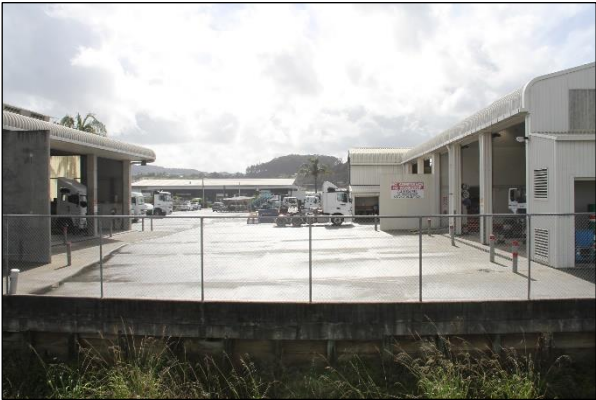
Southern view of yard
