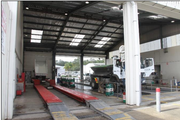
Truck inspection bay
