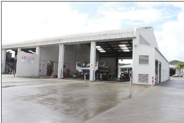
Truck inspection bay
