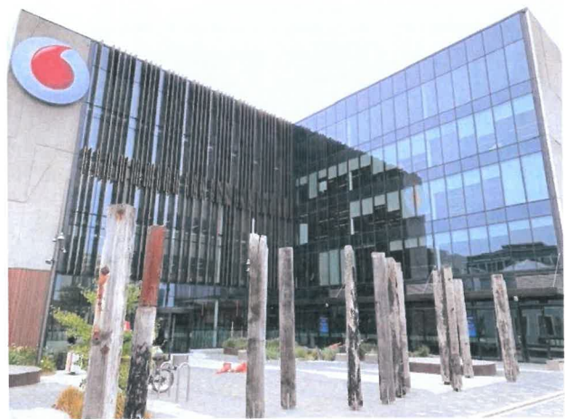
Exterior Tuam Street Frontage
