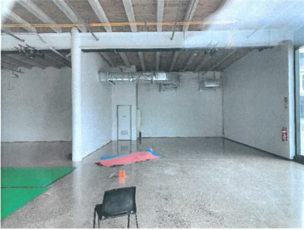
Ground Floor Retail Area
