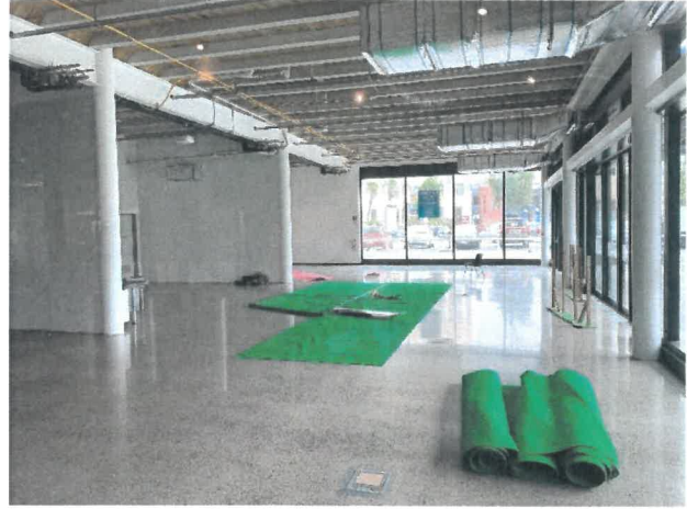
Ground Floor Retail Area
