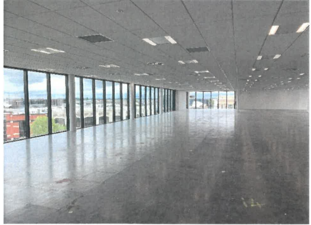
Level 4 Vacant Office Area
