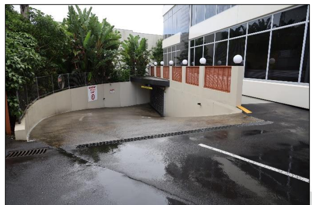
Basement carpark access
