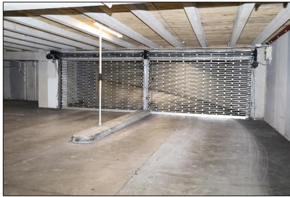
Basement parking security
