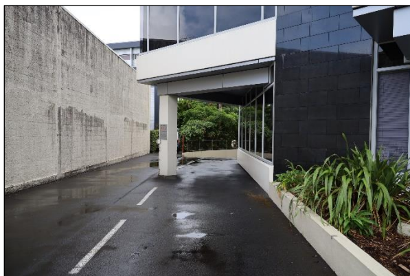
Basement carpark access
