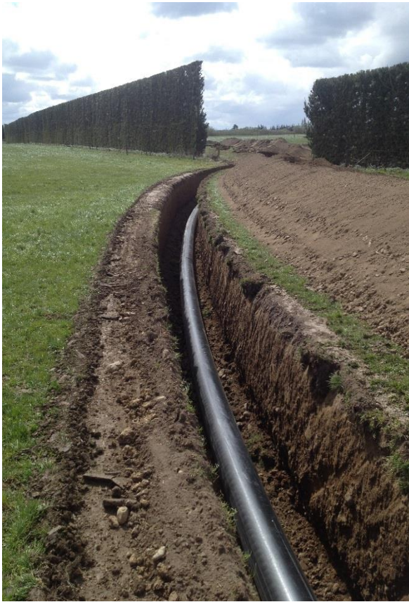
Example of HDPE pipe installation (Stage 1)
