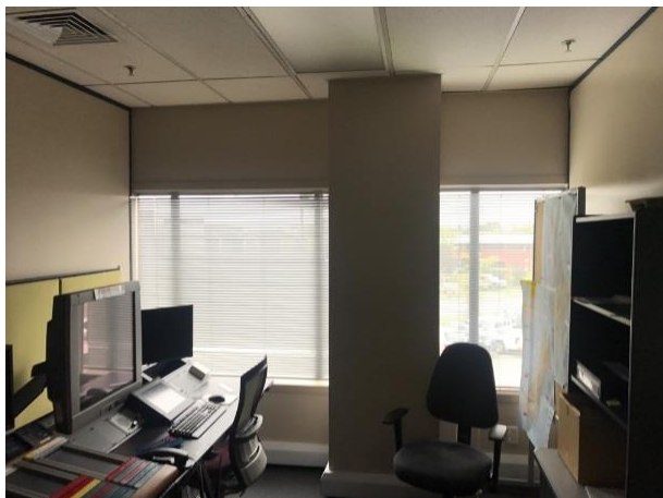
B2 – perimeter column
