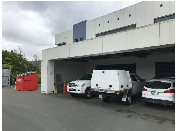
B2 – covered carport and garages
