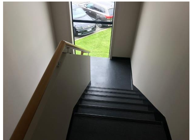
B2 – Internal fire escape stair
