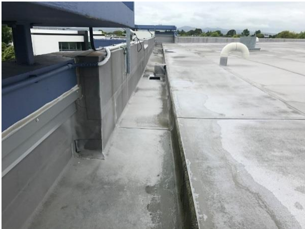
B2 – perimeter concealed gutter
