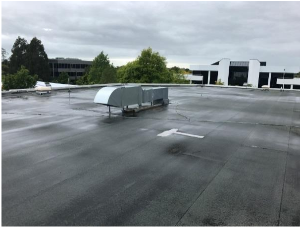
B1 - General view over roof
