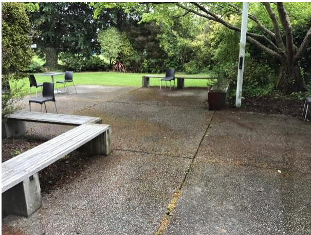
Hard standing to NW corner of B1.
