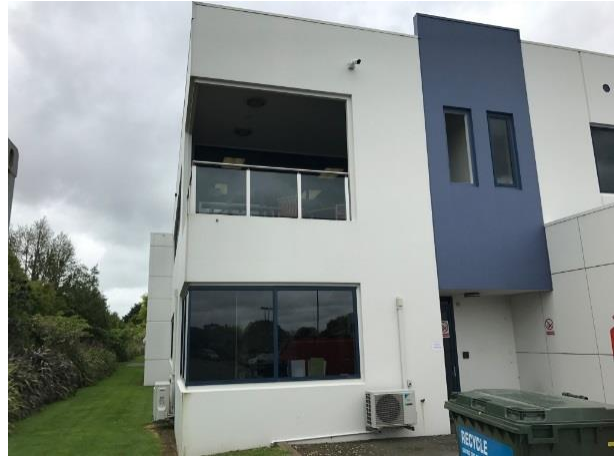
B2 – SW corner & semi enclosed deck area
