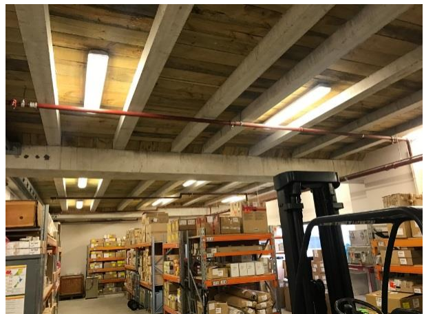
B2 – storage area to south end of building
