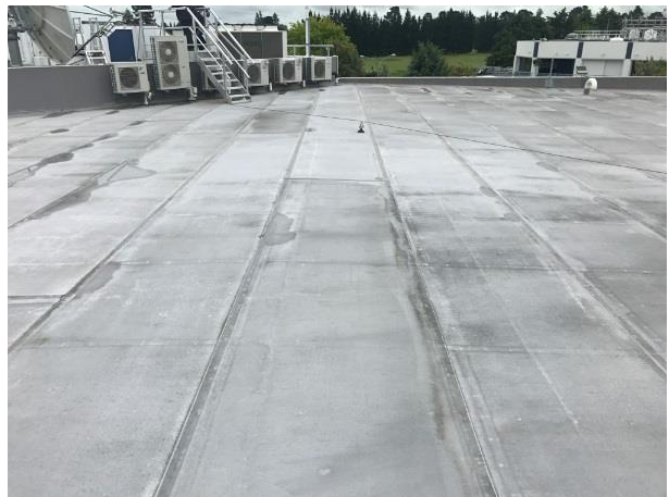
B2 - General view over roof to 2007 Ext
