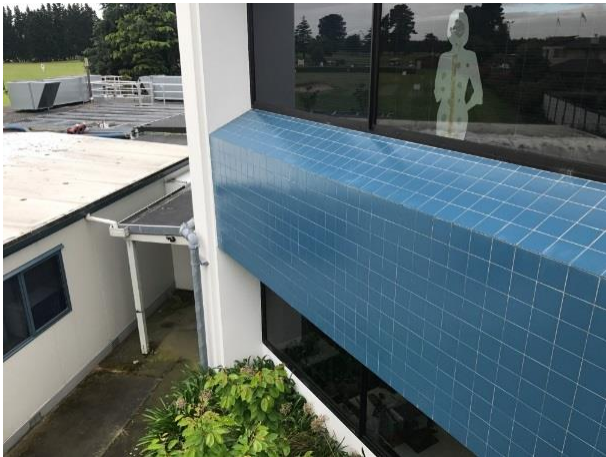
B1- Tiled concrete sections
