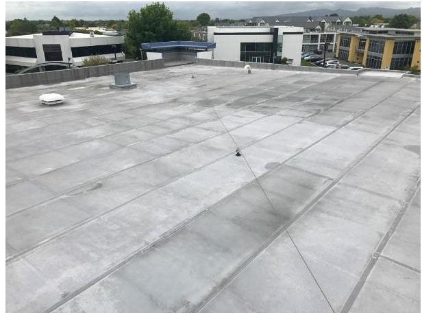
B2 - General view over roof to 2007 Ext
