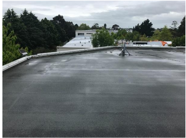
B1 - General view over roof
