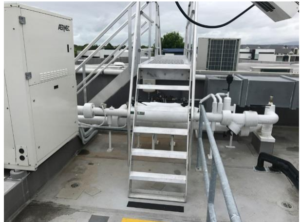
B2 – fixed stairs providing access over roofs
