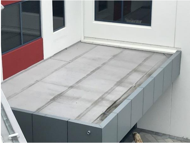
B2 – flat roof over entrance lobby.
