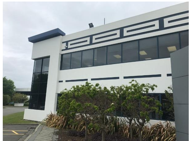
B2 - North elevation of 2007 extension
