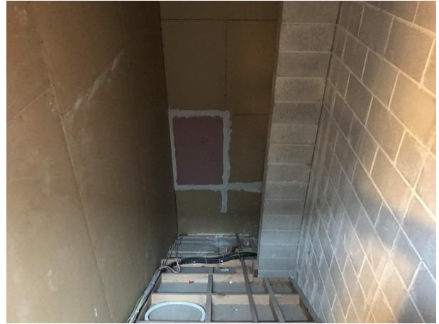
B1- Internal blockwork wall & pier
