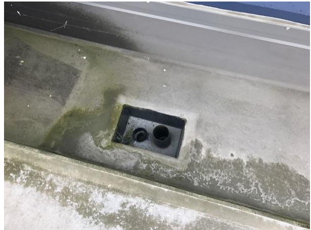
B2 – standard drainage outlet
