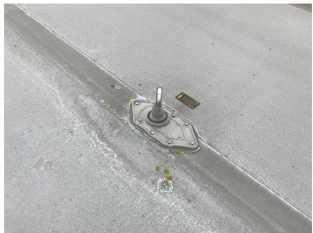
B2 – typical anchor point
