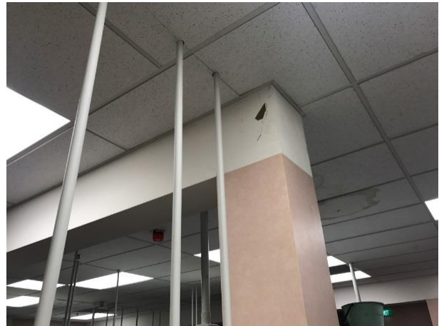
B1- Internal concrete goalpost support
