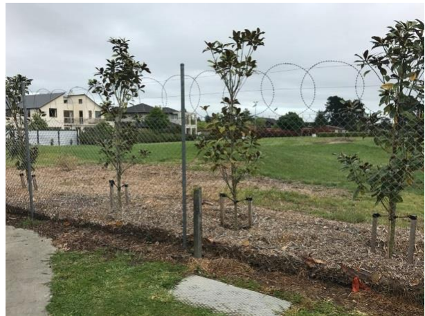
Chain-link perimeter fence & razor wire.
