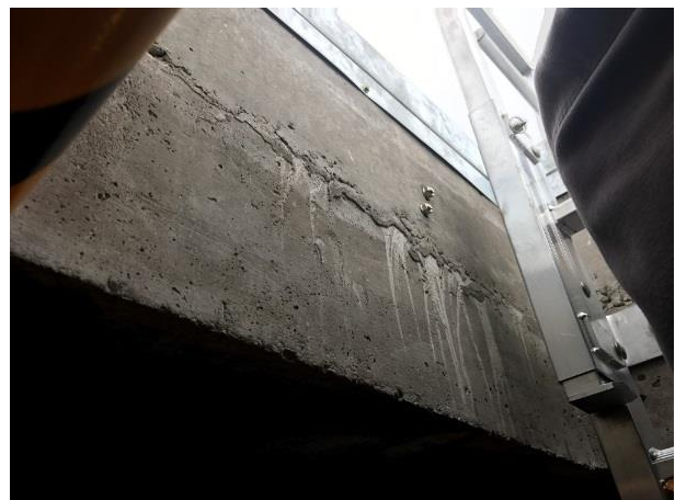
B1- Concrete roof slab
