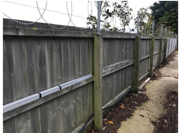
Timber perimeter fence.
