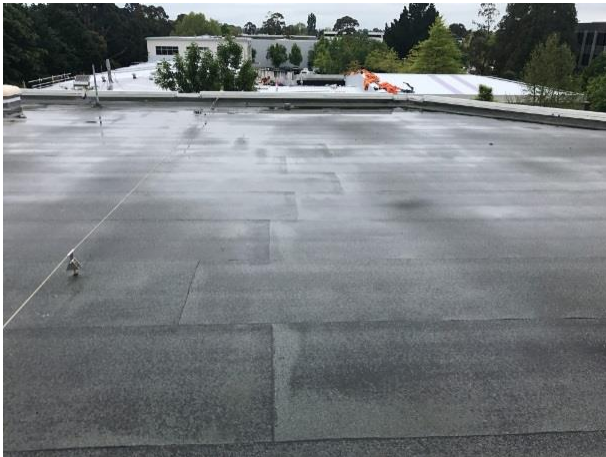
B1 - General view over roof
