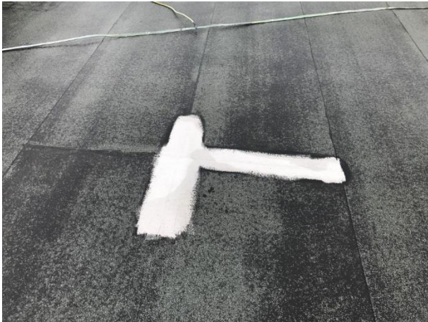
B1 – Liquid applied patch repair.
