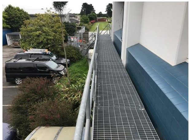
B1 – New metal external fire escape stair
