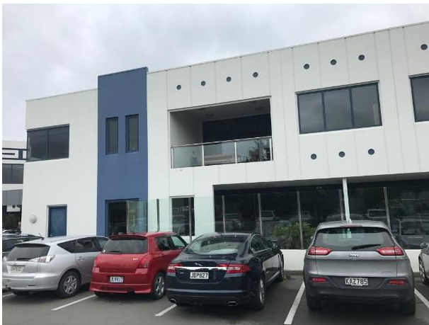
B2 – North elevation of original 1992 build
