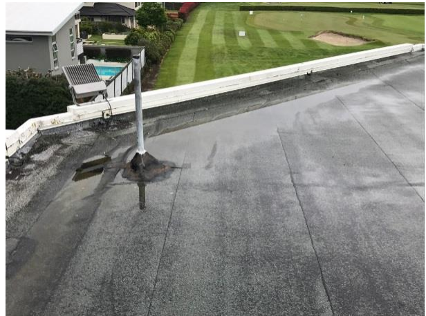
B1 - General view over roof
