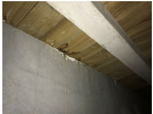
1.58. Basement - Timber formwork noted to be stained and displaying evidence of moisture ingress
