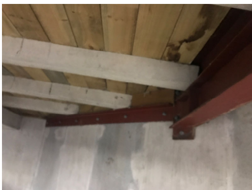
1.53. Basement - Timber formwork noted to be stained and displaying evidence of moisture ingress
