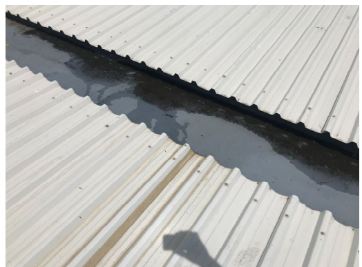
1.12. Plant discharging condensate water into gutters
