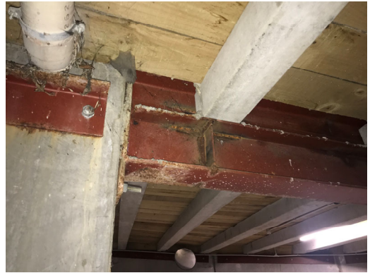
1.56. Basement - Steel noted to be corroding adjacent to stained timber formwork
