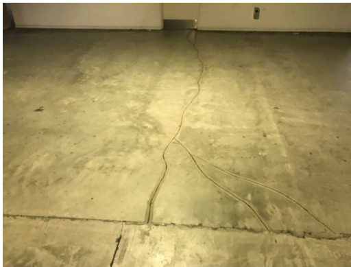
1.57. Basement - Cracking noted to car park surfaces – cracks appear to have been filled in and repaired
