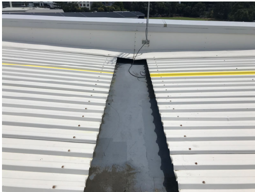
1.3. View of gutter membrane
