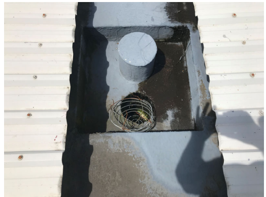
1.10. Sump gutters within valley gutters
