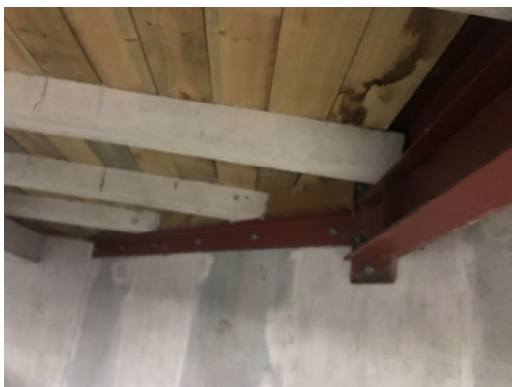
1.59. Basement - Timber formwork noted to be stained and displaying evidence of moisture ingress
