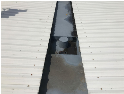
1.9. pWater inlet within valley gutters
