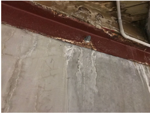
1.55. Basement - Steel noted to be corroding adjacent to stained timber formwork
