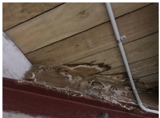
1.54. Basement - Steel noted to be corroding adjacent to stained timber formwork
