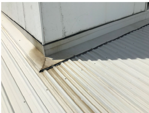
1.11. Apron flashing to plant screen
