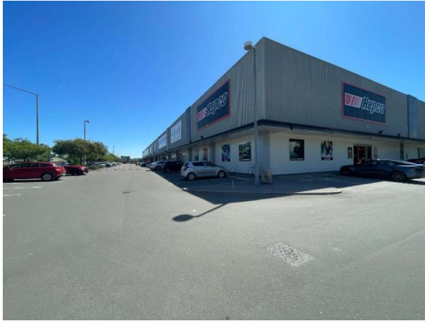
Repco Exterior and Car Parking
