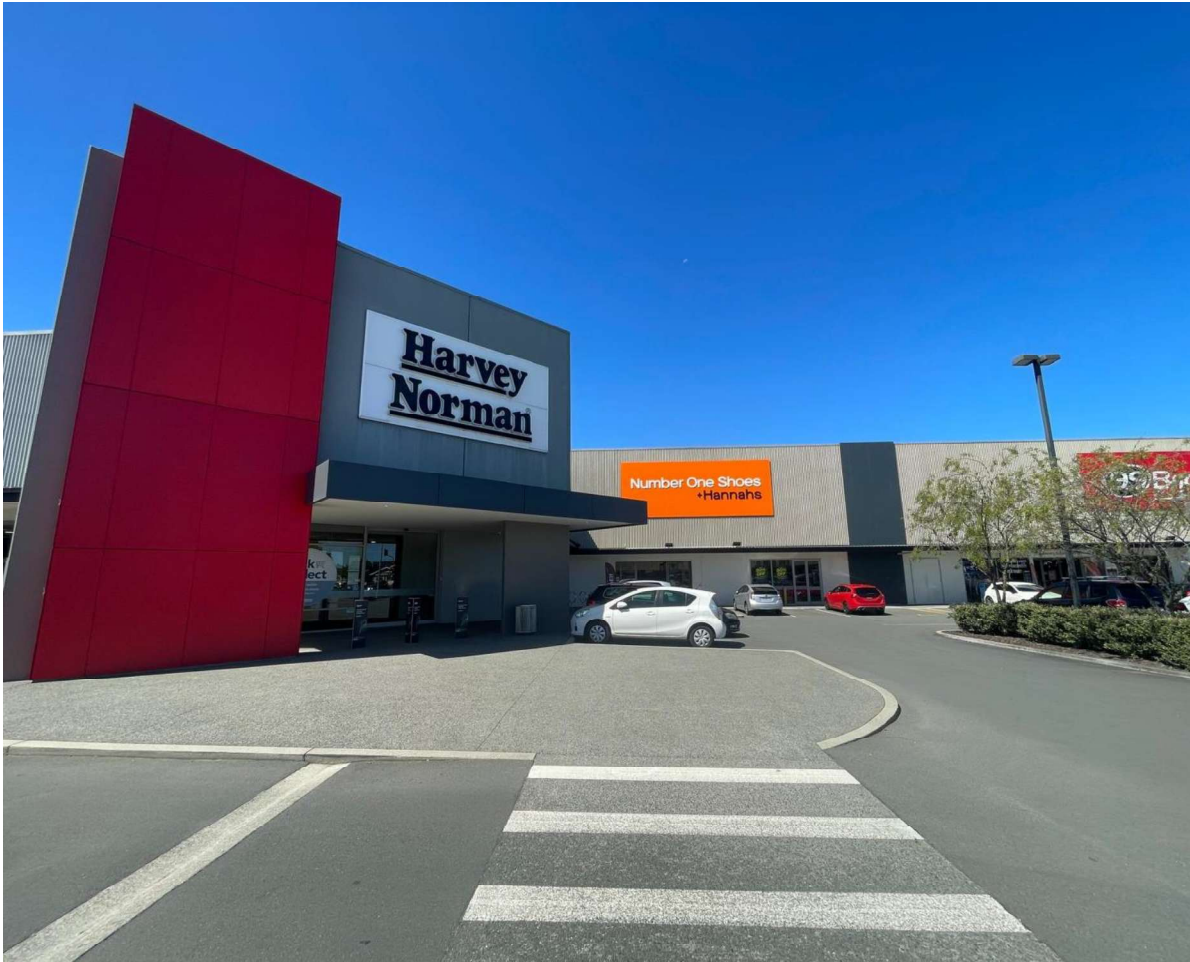
Photo from Physical Inspection – Source JLL
