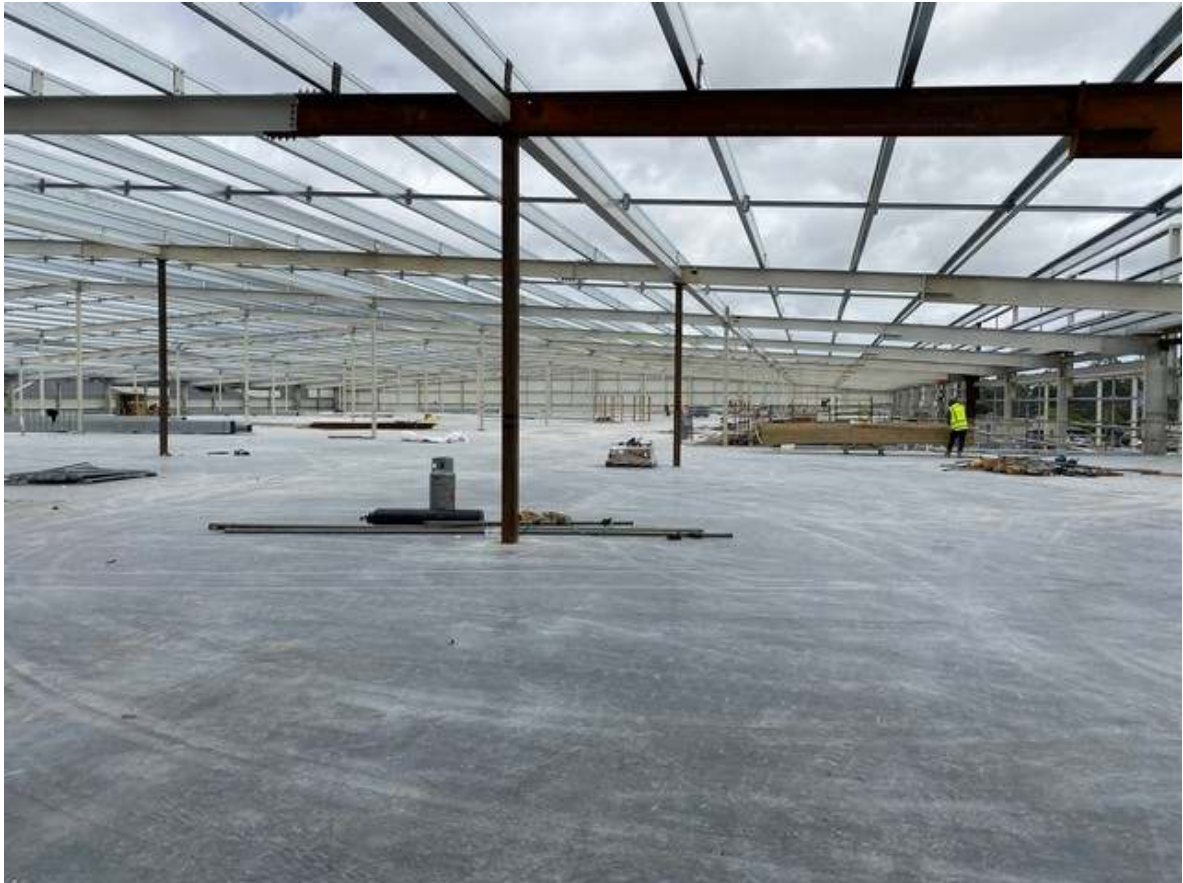
Construction continues November 2019
