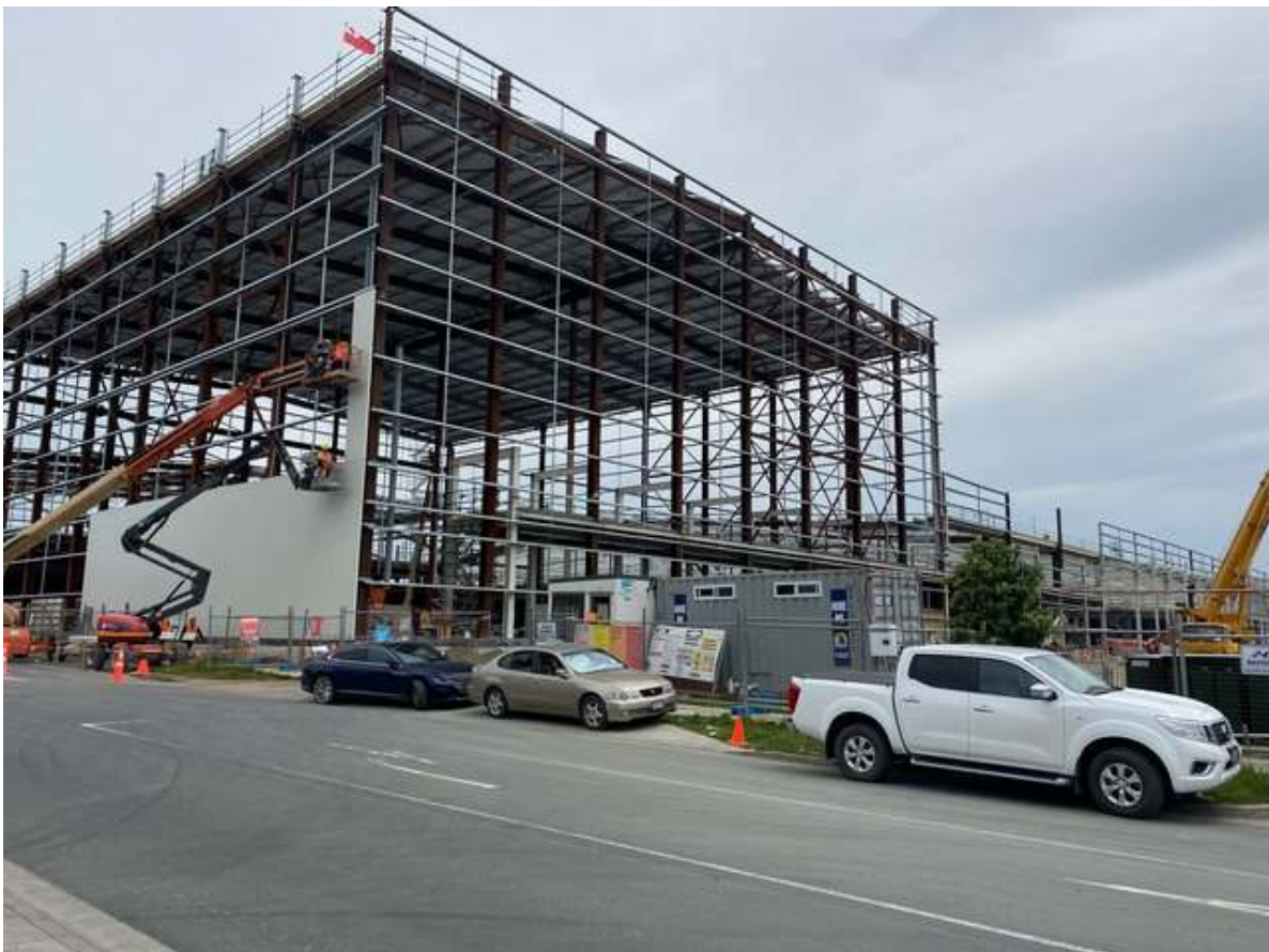
Construction on walls November 2019
