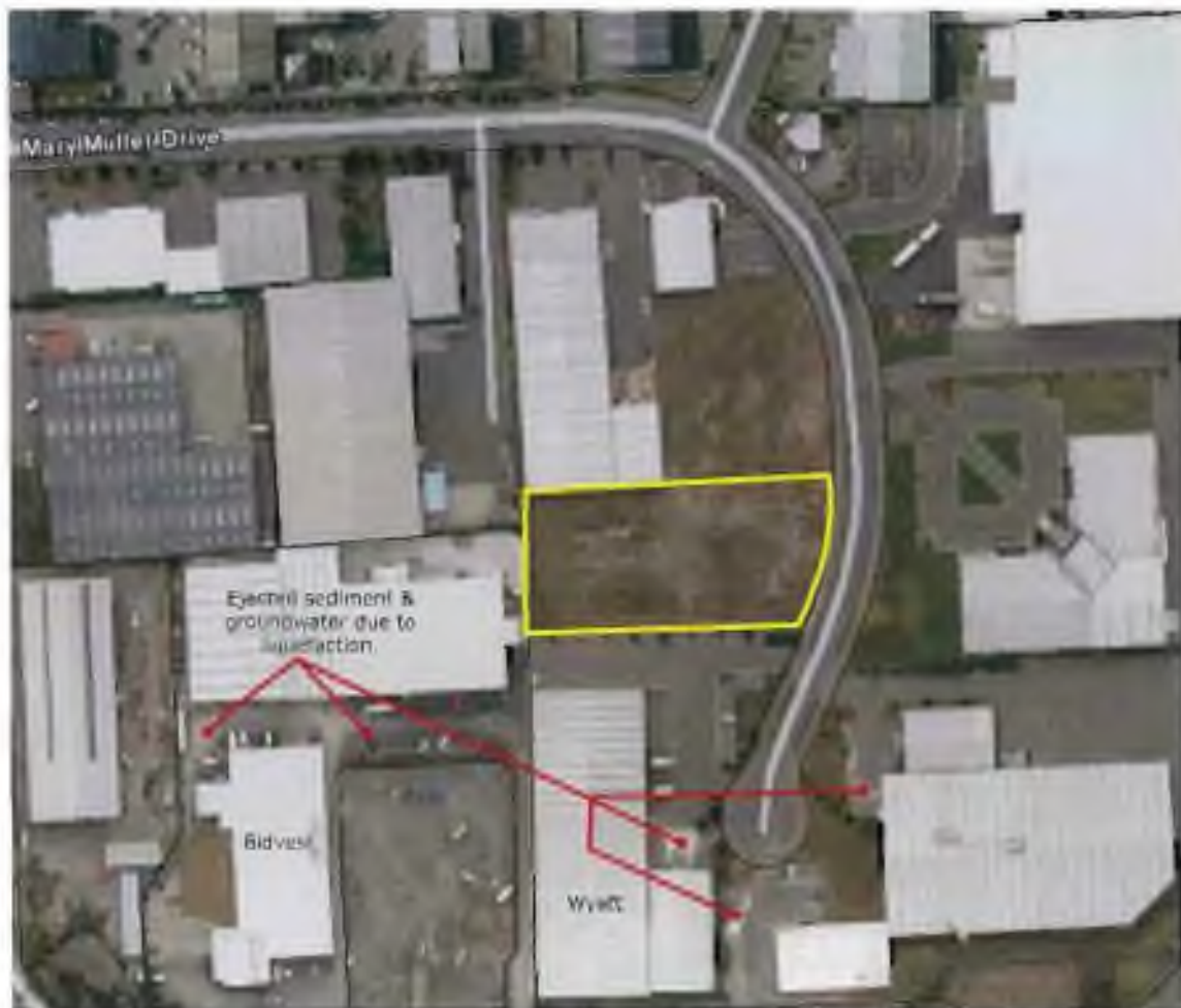
Land Damage on Mary Muller Drive. The approximate site boundary is in yellow. Source: Canterbury Recovery, Project Orbit. Photographs taken 24 February 2011.
