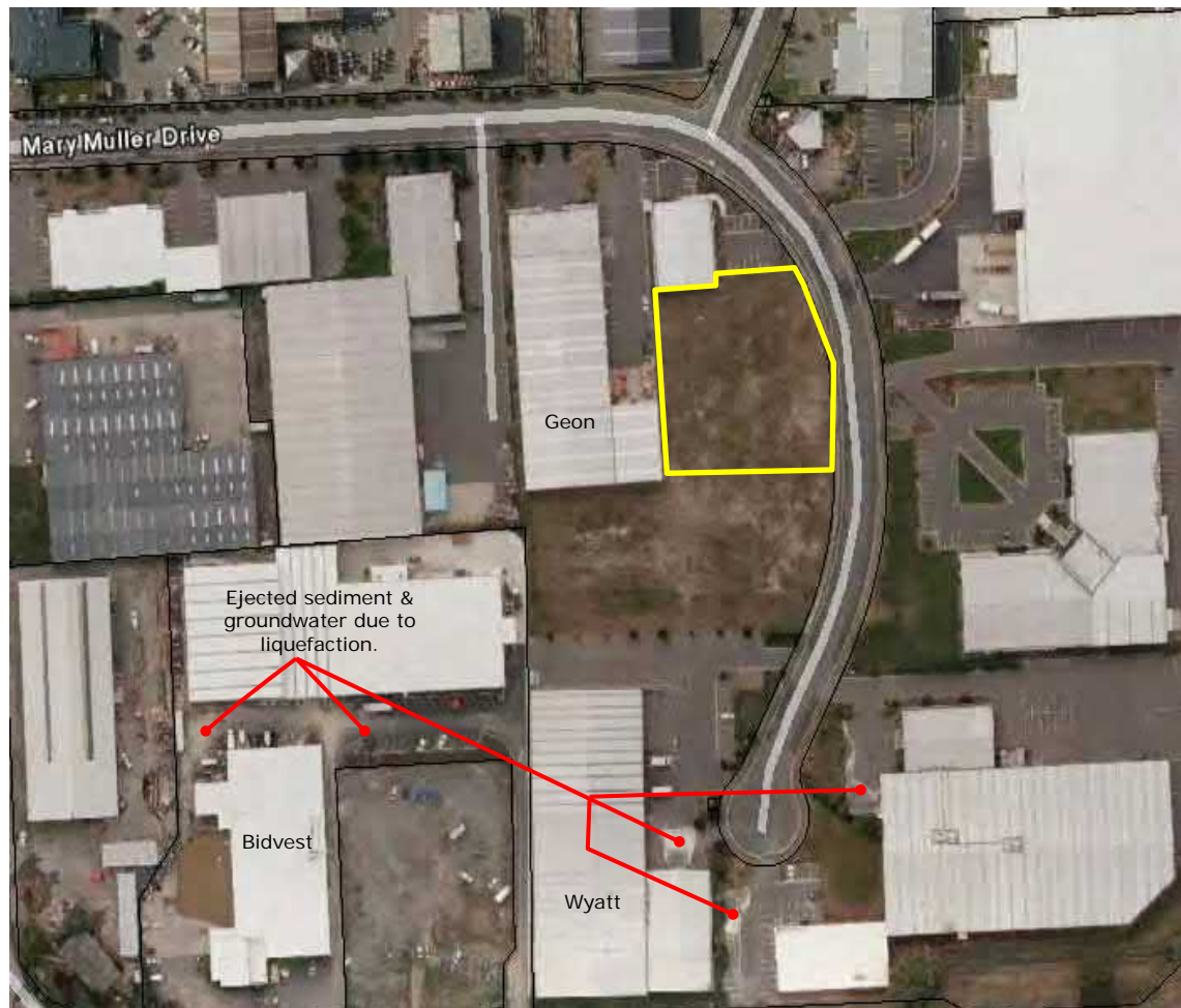
Land Damage on Mary Muller Drive. The approximate site boundary is in yellow. Source: Canterbury Recovery, Project Orbit. Photographs taken 24 February 2011.
