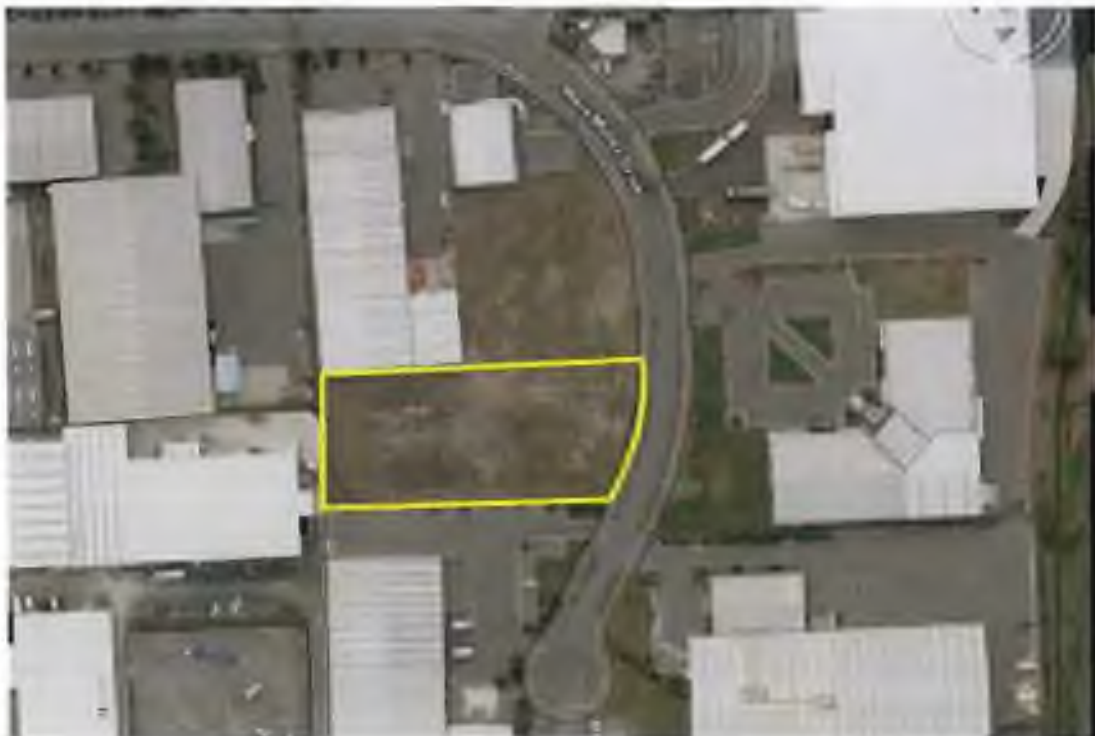
Diagram 1: Site location plan (approximate boundary in yellow), (source: Canterbury Recovery, Project Orbit, photo from 24 February 2011).
