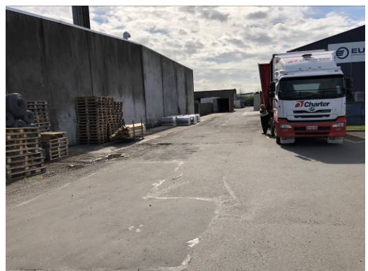
1.26. Cracking and historic repairs to yards
