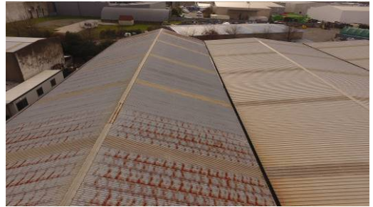
1.2. View of corroded Roof fixings to Bay 1
