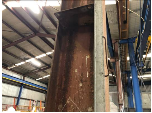
1.22. Corroded columns noted
