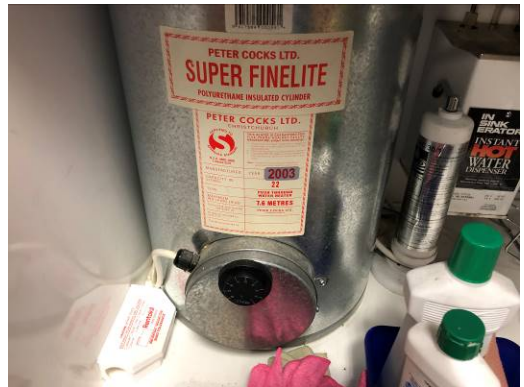
1.30. Typical hot water cylinder
