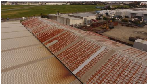
1.1. View of corroded Roof fixings to Bay 1
