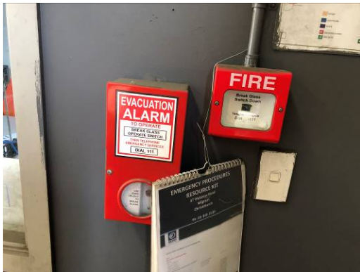
1.29. Typical wall mounted fire switching
