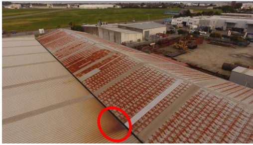
1.1. Location of heavy corrosion to Roof Bay 2
