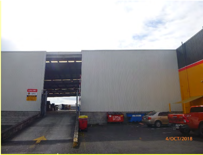
Photograph 25 Recco Open Warehouse.
