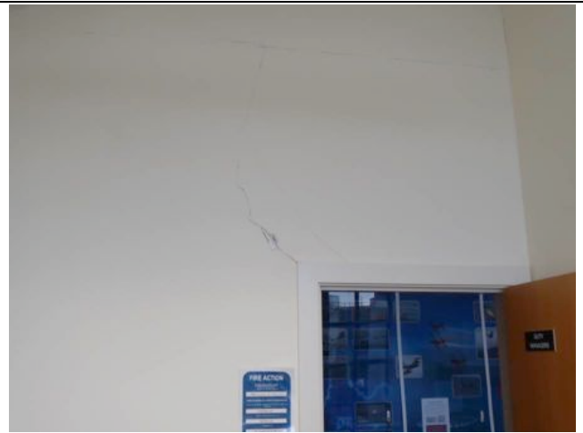
Photo 6: Typical internal lining damage
