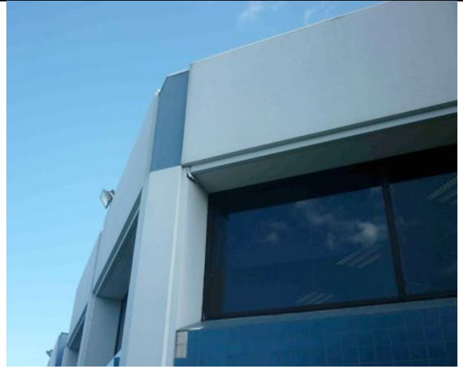
Photo 2: Spandrel / column cladding crushing
