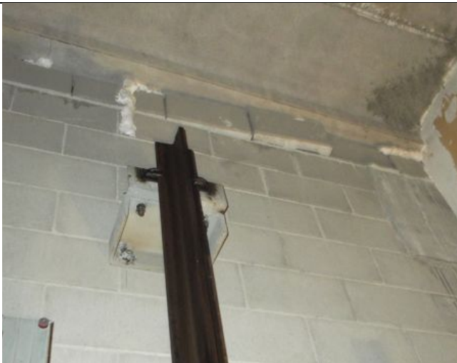
Photo 7: Lift shaft Blockwall – loose blocks at top
