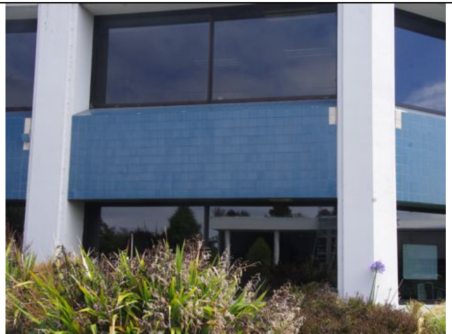
Photo 10: Further external tile cladding damage
