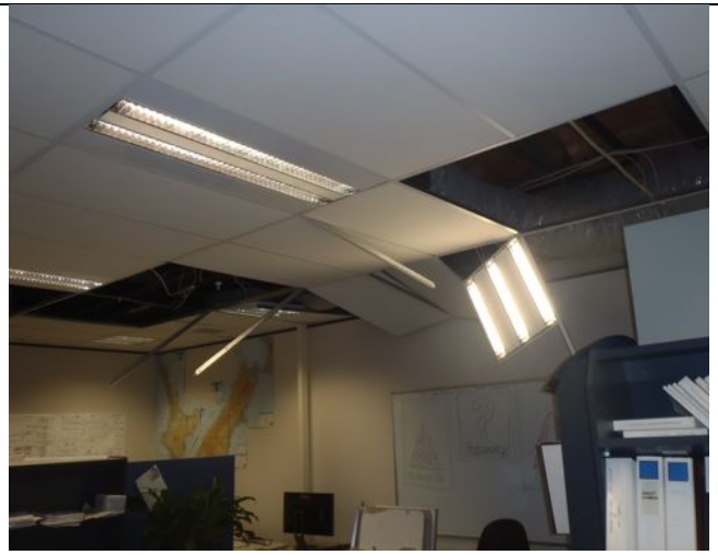
Photo 8: Typical suspended ceiling damage at Airways
