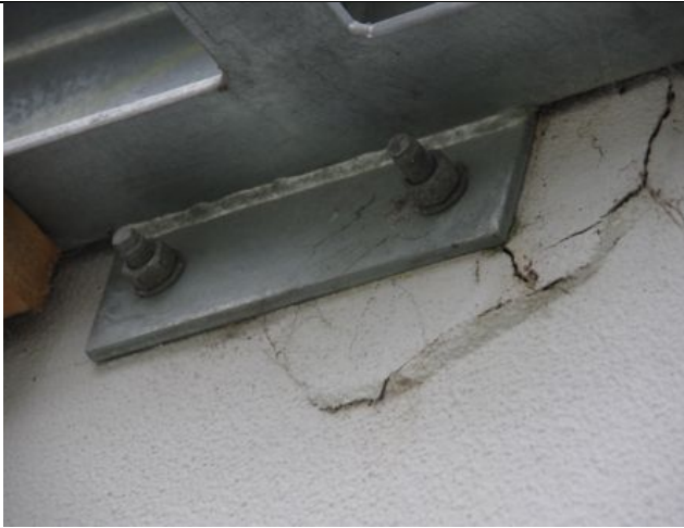
Photo 5: External walkway spalling of concrete at joint
