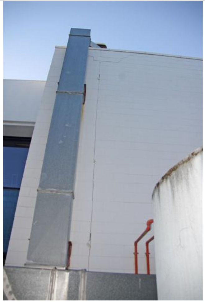
Photo 4: Western blockwall cracking
